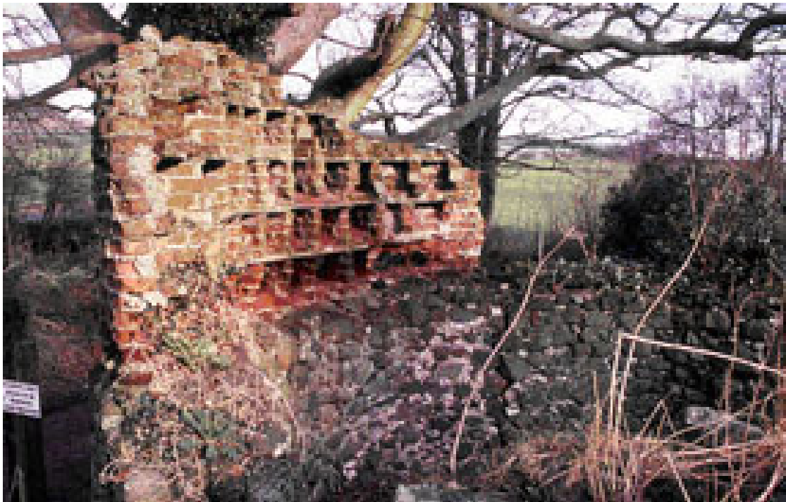
Plate Eleven: Details of the later brick built dovocote in the northeastern bastion (looking northeast).
