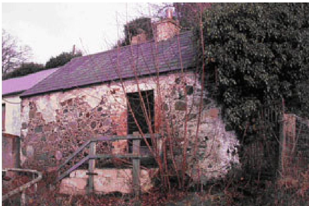
Plate Eighteen: Stone built single storey outbuilding with a single central, brick built chimney (looking northeast). As the outbuilding is built on the same alignment as Kilroot House it is possible that it was converted into its current form from the western part of Kilroot House.
