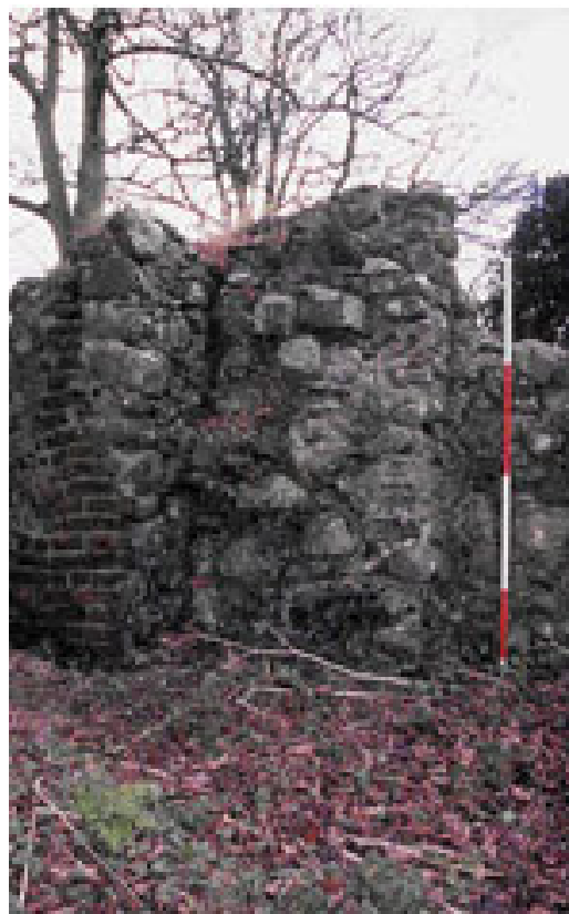
Plate Twelve: Short stub of an apparently earlier wall incorporated into the fabric of the northeastern circular bastion (looking southeast).
