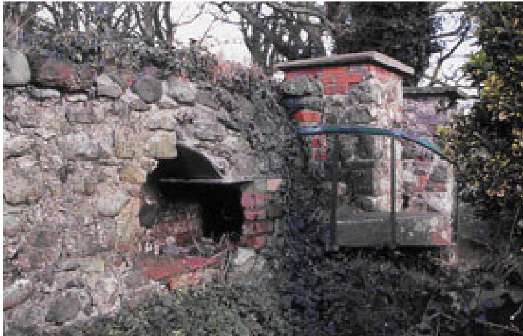
Plate Thirteen: Brick and slate built alcove, set into the graveyard's northern retaining wall, in which the sexton would have stored his tools (looking northeast).
