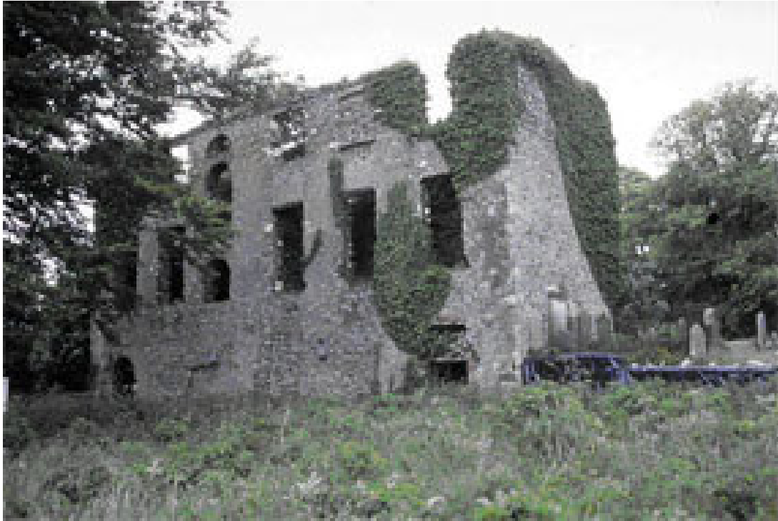
Plate One: The south-facing side of Kilroot House.
