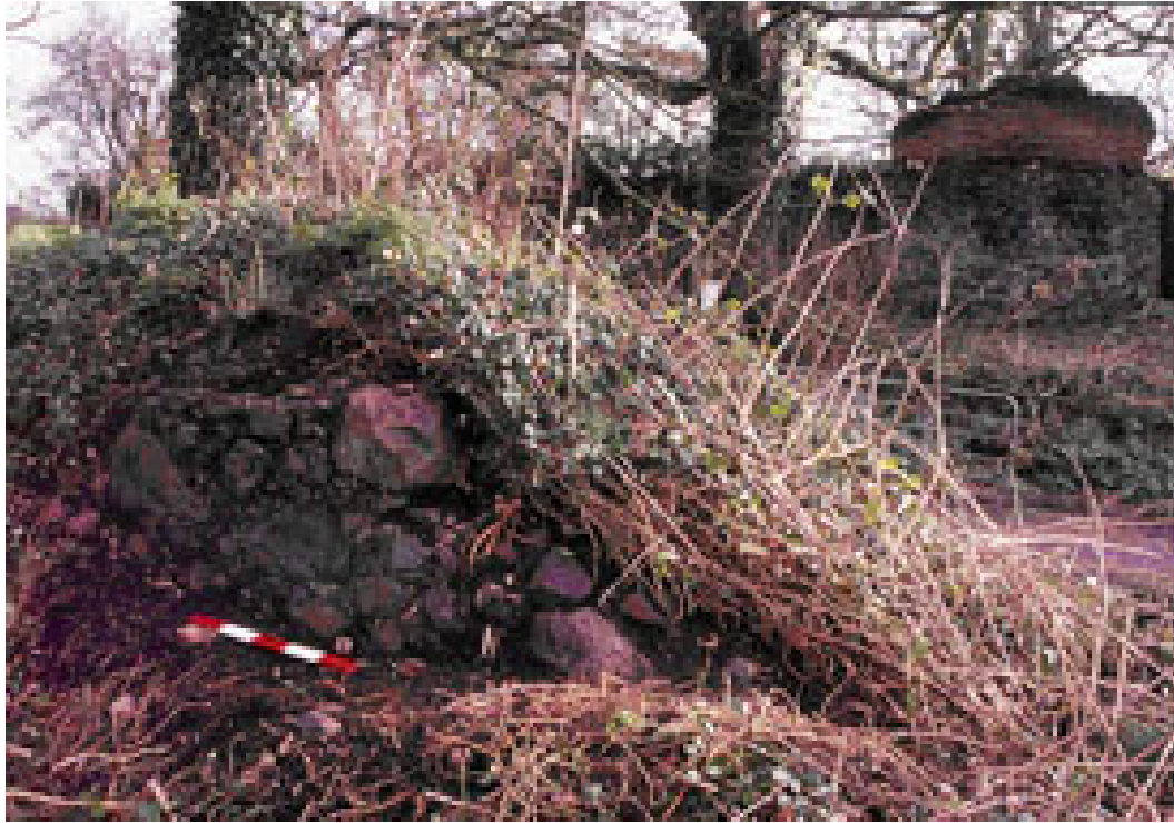
Plate Fifteen: Surviving length of wall within outlying triangular-shaped earthwork to the north of modern graveyard (looking southeast).
