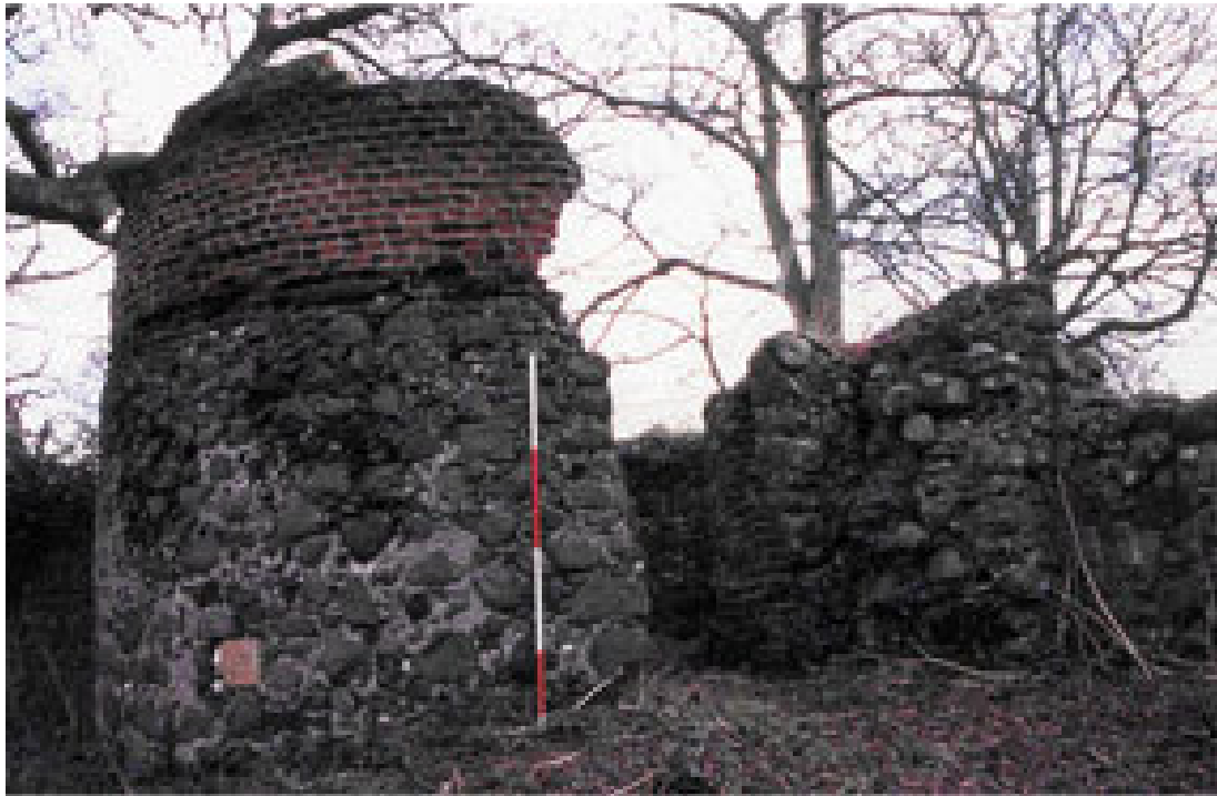
Plate Ten: Northeastern bastion (looking south). Note the remains of the later brick built dovocote and the pre-existing length of walling immediately to the west of the bastion.
