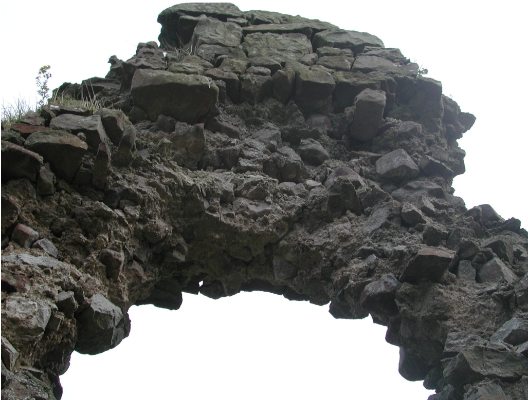
Plate One: Apex of eastern gable of church (looking east)
