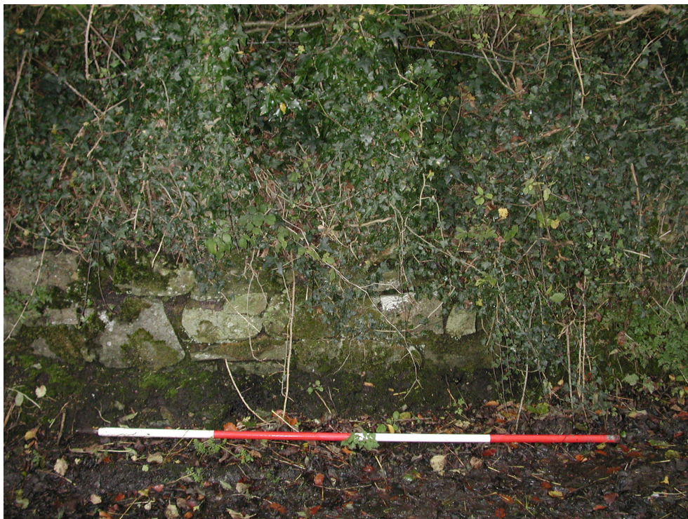
Plate Five: Mortared stones in wall of graveyard boundary (looking north)
