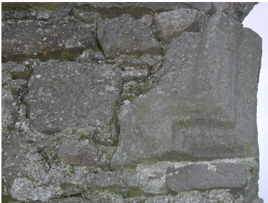
Plate Two: Relict window tracery exterior of eastern gable of church (looking west)
