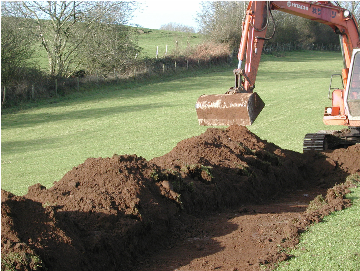
Plate 1: Excavation of Trench 2 showing utilization of toothless “sheugh” bucket.
