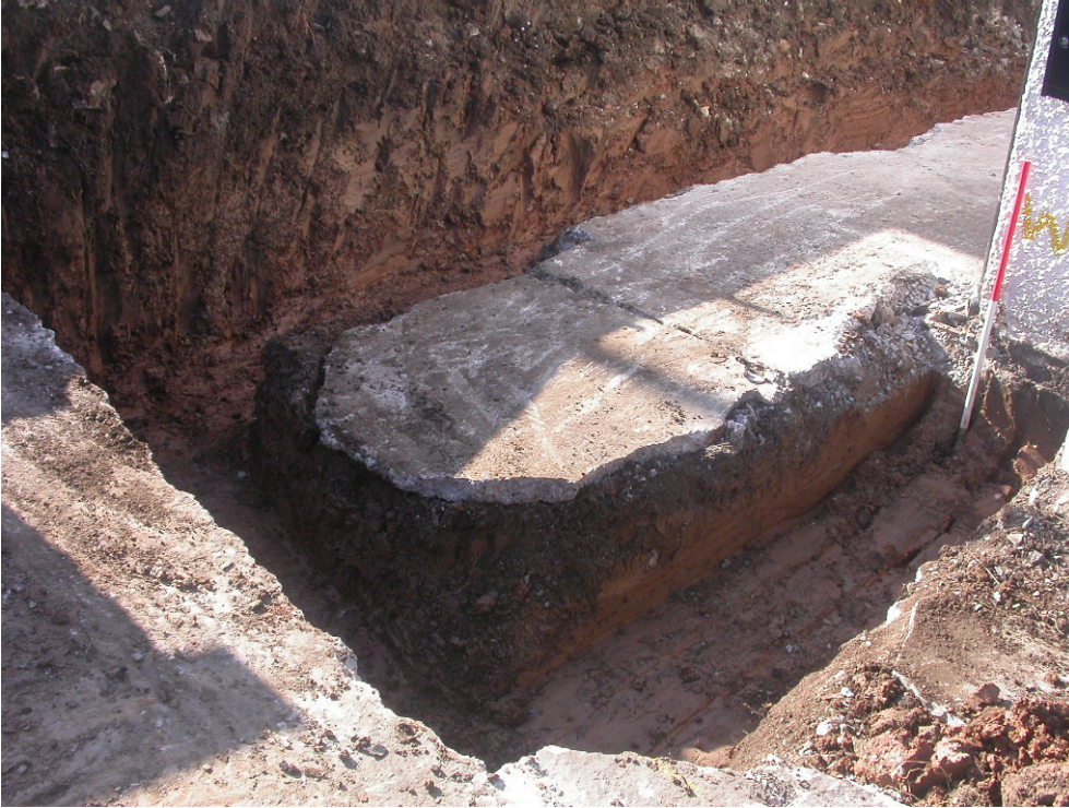
Plate 3: View of excavated foundation trench from south-east.
