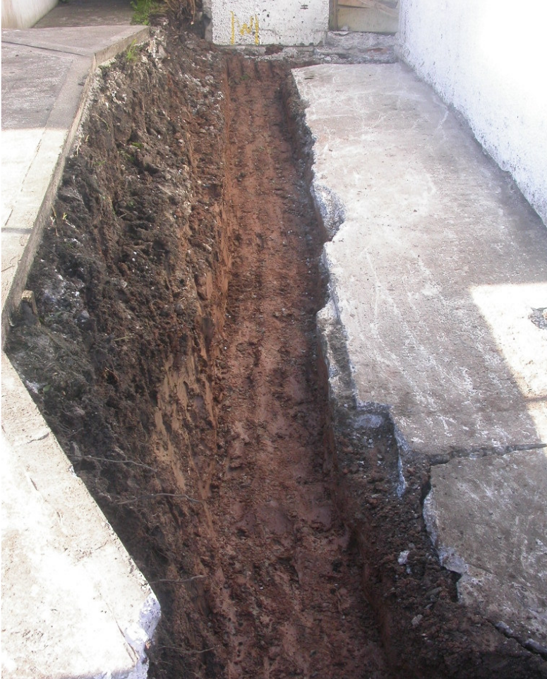
Plate 4: View of excavated foundation trench from south.
