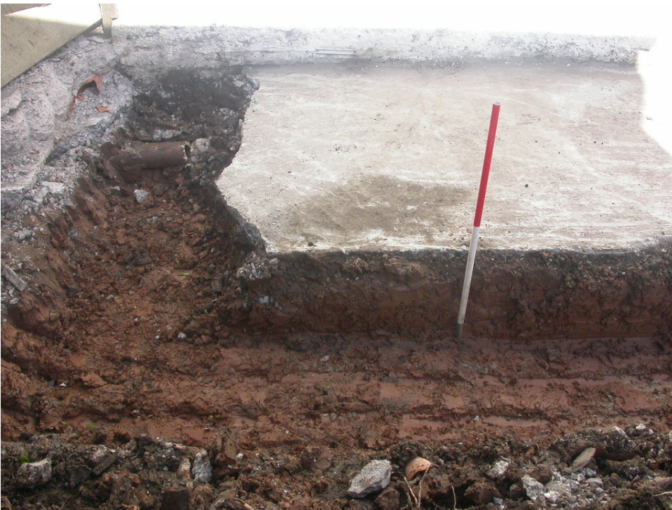
Plate 2: View of site from west after excavation of foundation trench.
