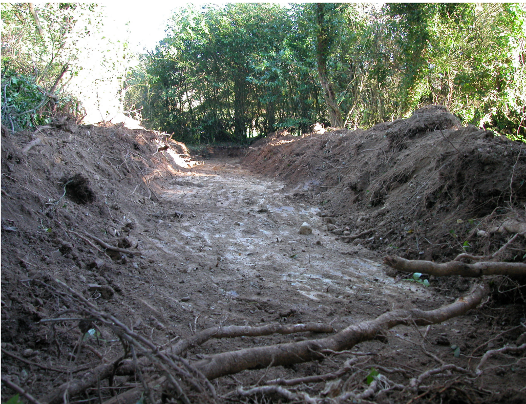
Plate 4: Trench 1, looking north-east.
