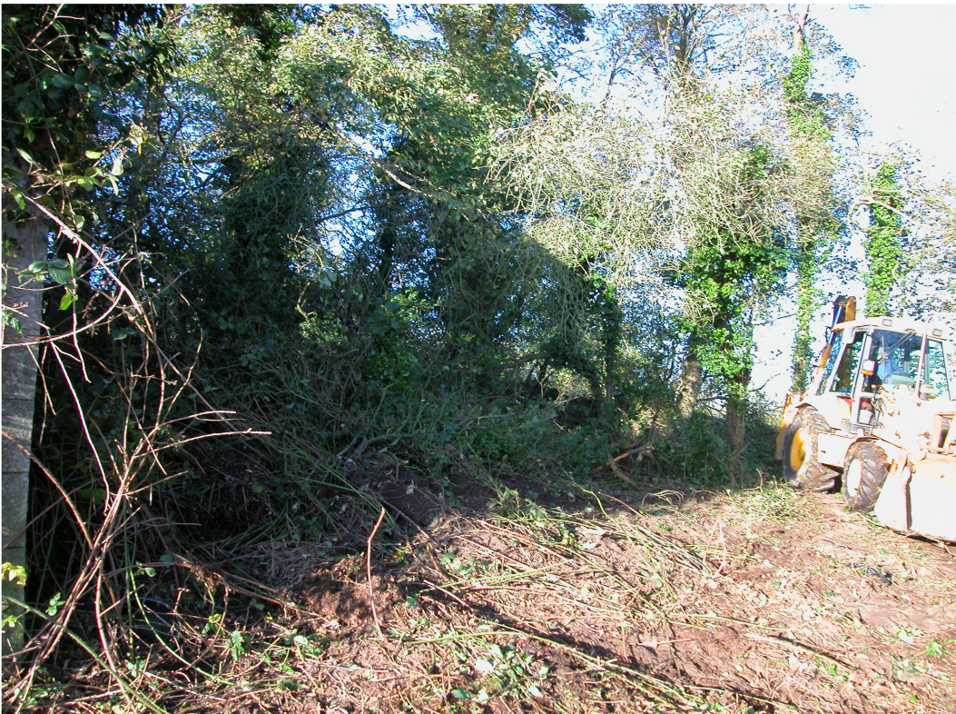
Plate 2: Unexcavated area along south-west edge of site.
