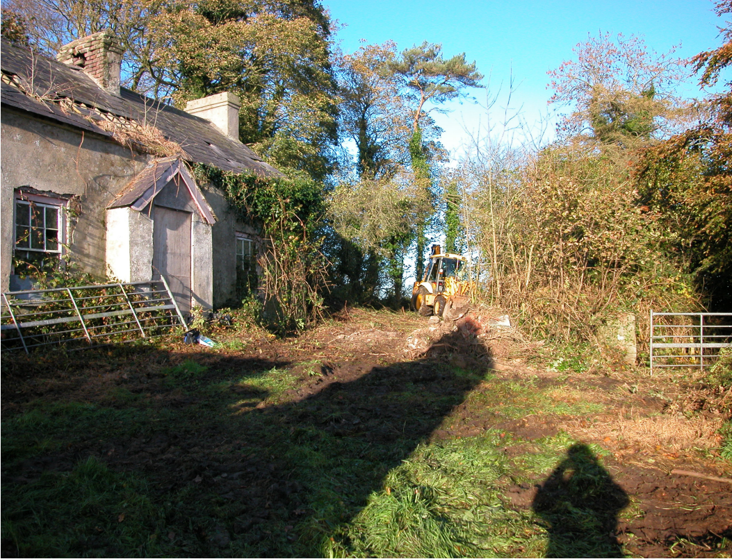
Plate 1: View of site with derelict dwelling, looking north-west.
