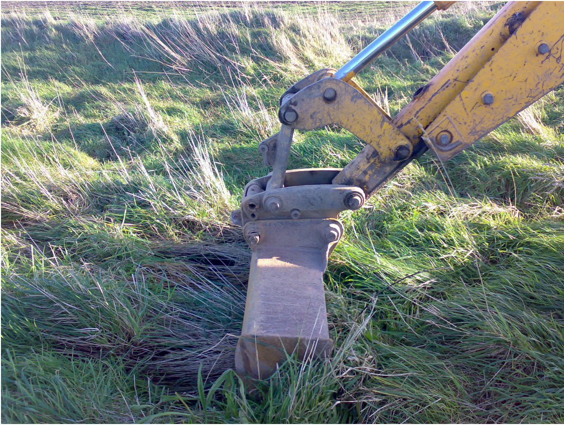
Plate 1: Excavation of Trench One, looking East
