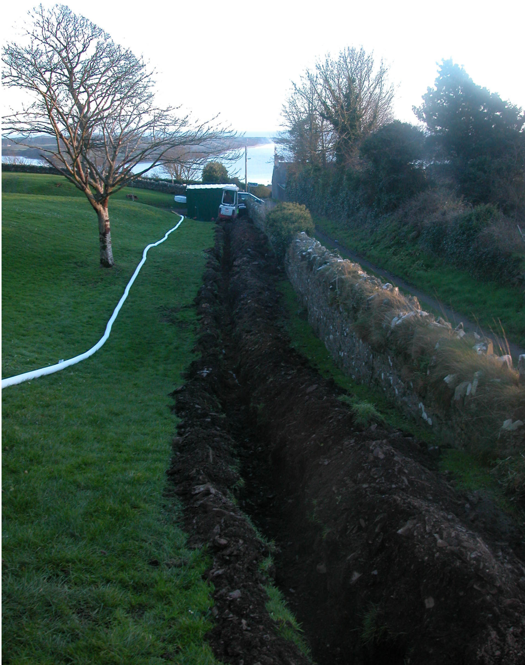
Plate 5: Trench 2, looking south-east.
