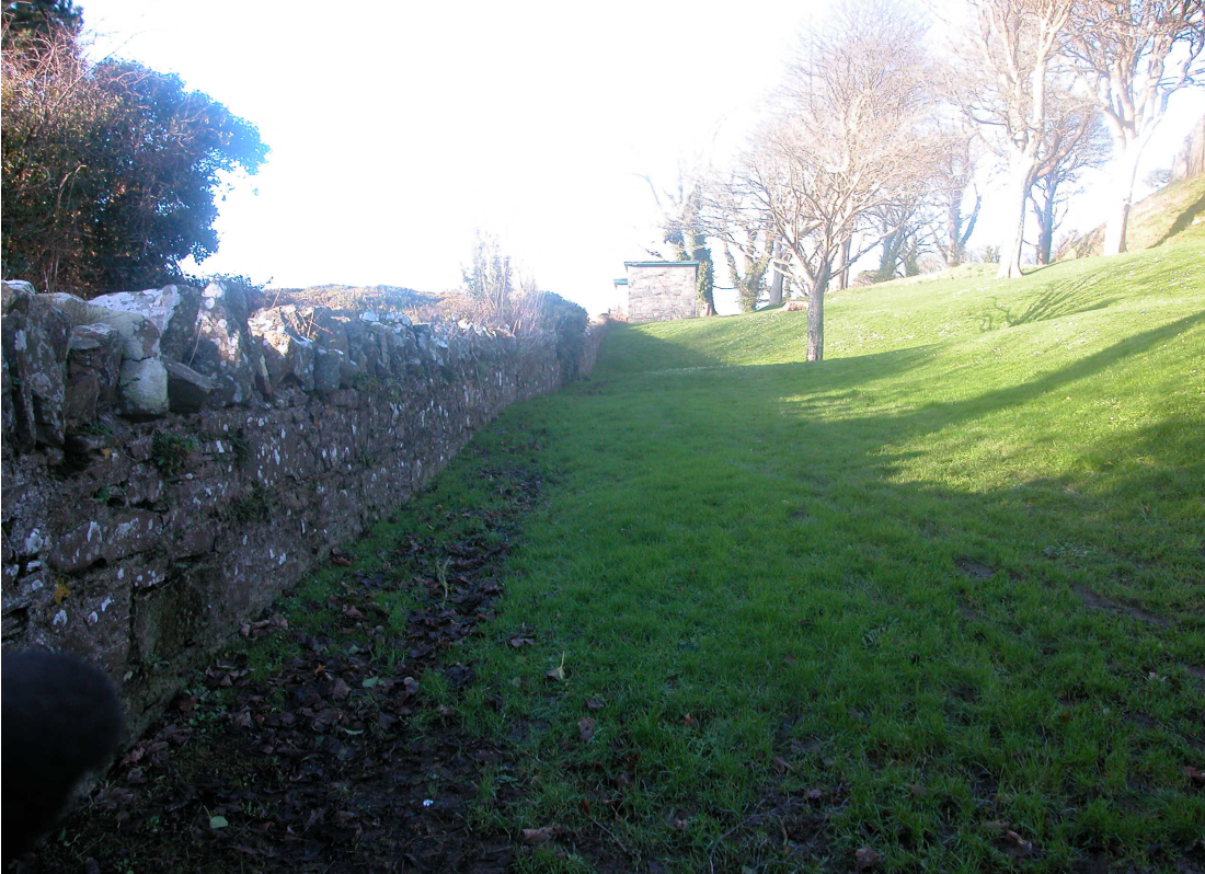
Plate 3: Boundary wall looking north-west towards toilet block.
