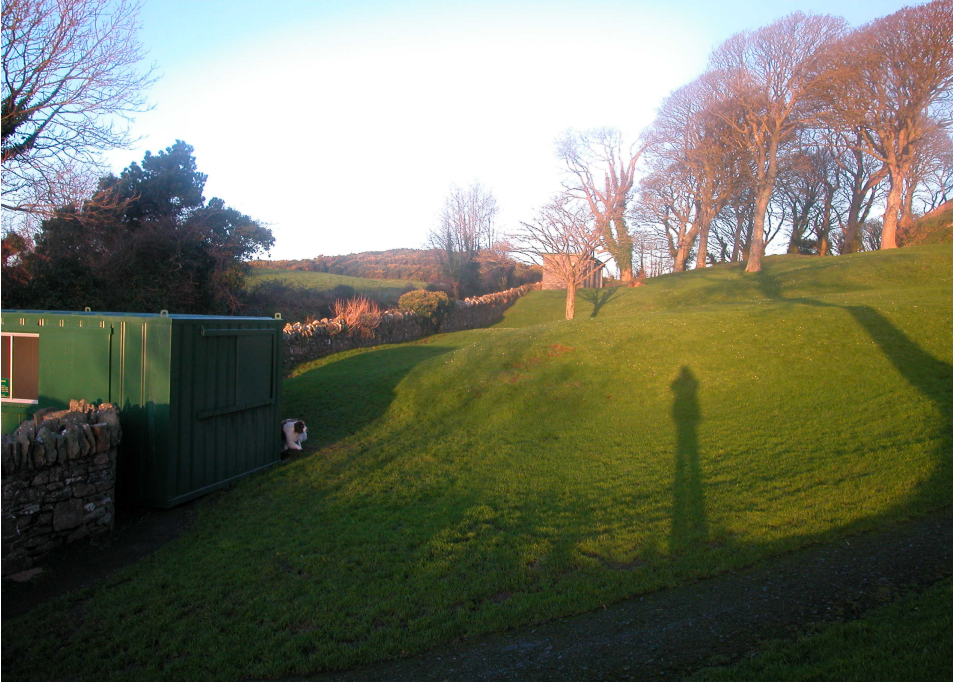
Plate 1: Photo showing new portacabin, boundary wall and toilet block, looking north-west.
