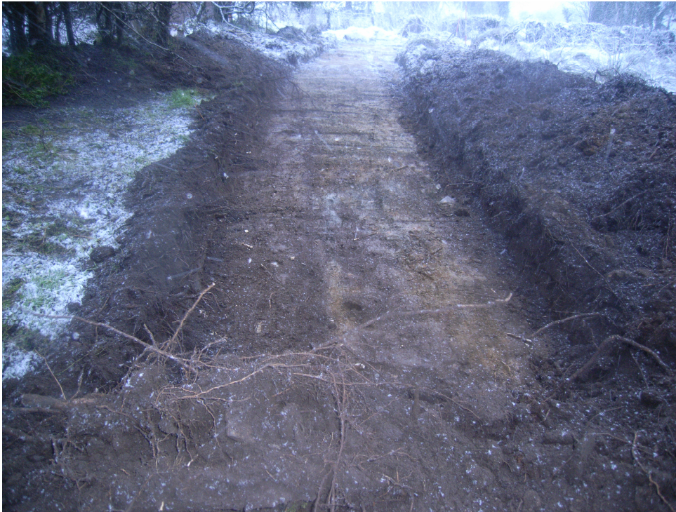
Plate 1: Trench One, following excavation to subsoil, looking north-east.
