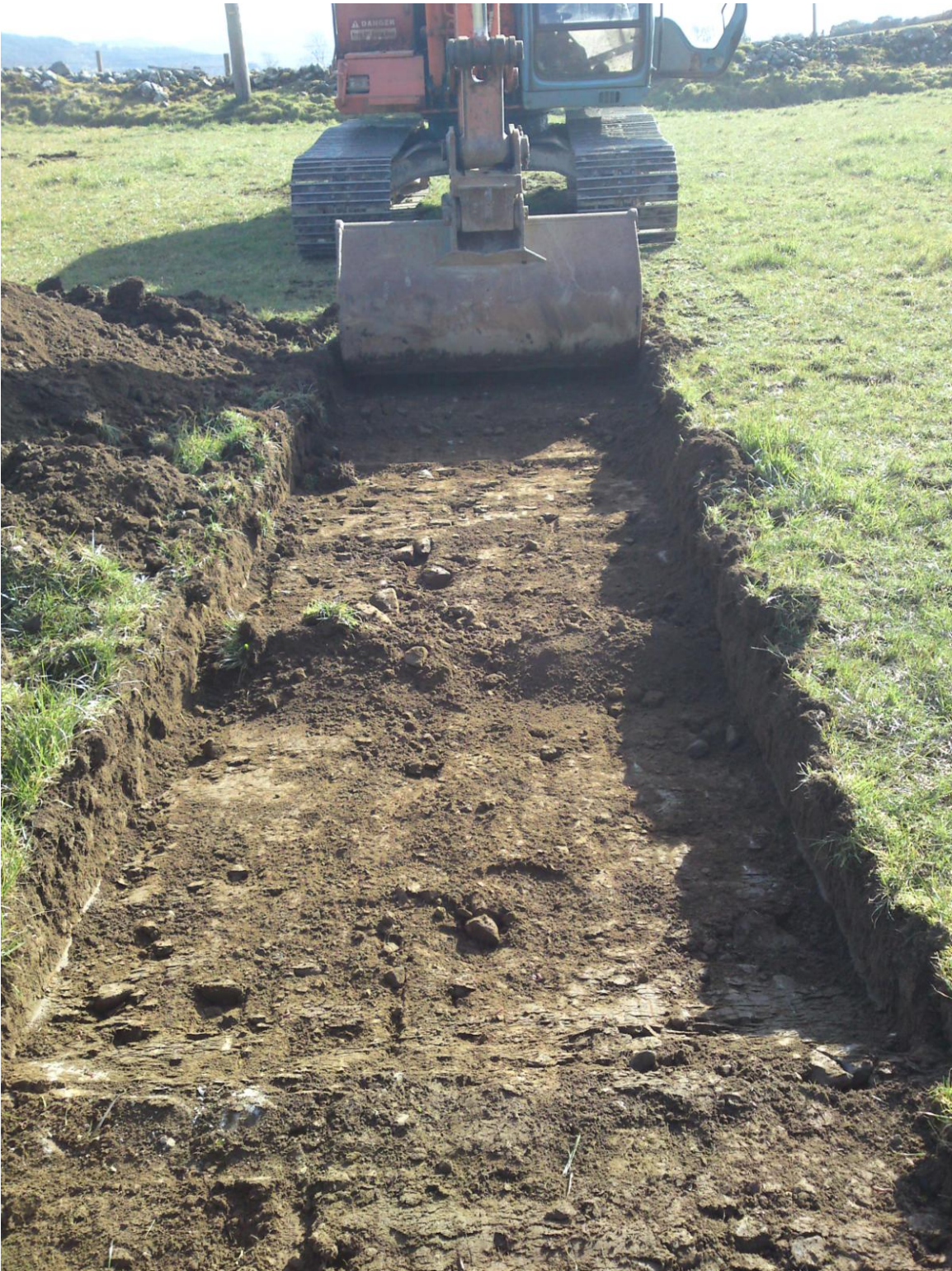
Plate 2: Mid excavation shot showing the excavation of Trench One to the surface of the natural subsoil (Context No. 102), looking north-west.
