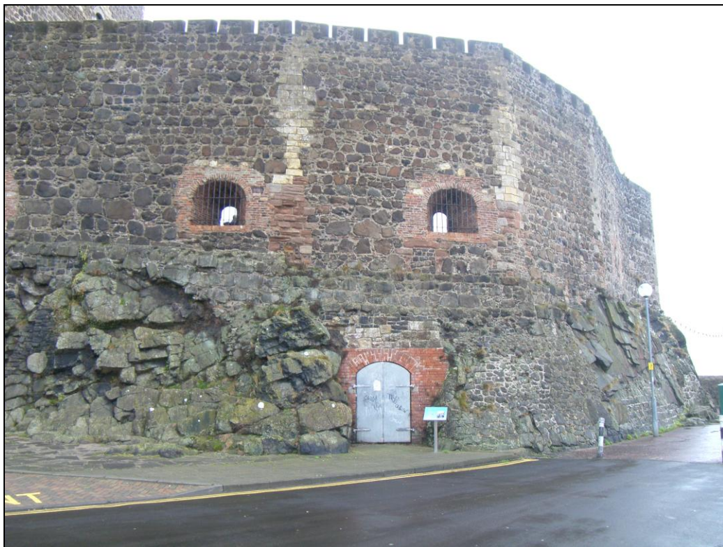
Plate 08: View of external entrance to access tunnel, looking south-east
