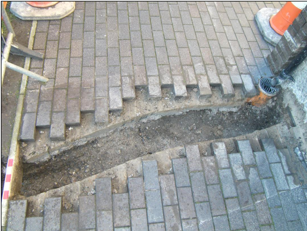
Plate 04: Trench 2: post-excavation view, looking west
