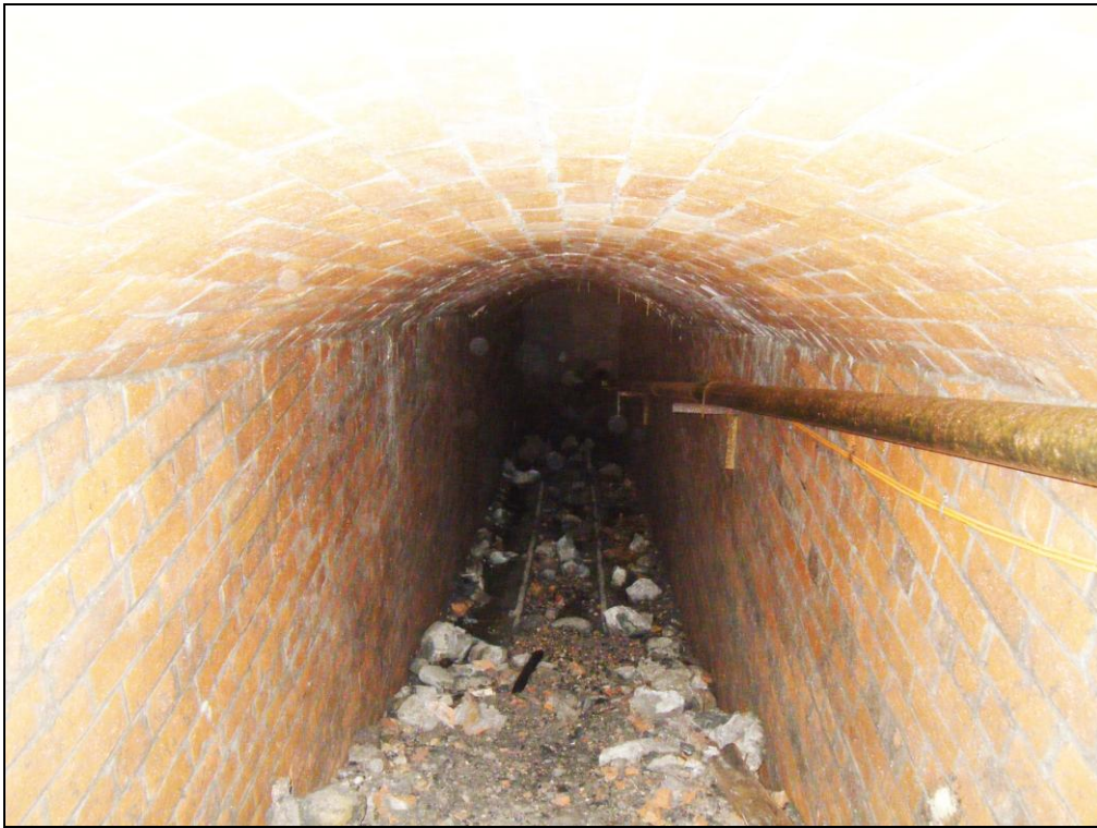
Plate 07: View of interior of access tunnel, looking north-west
