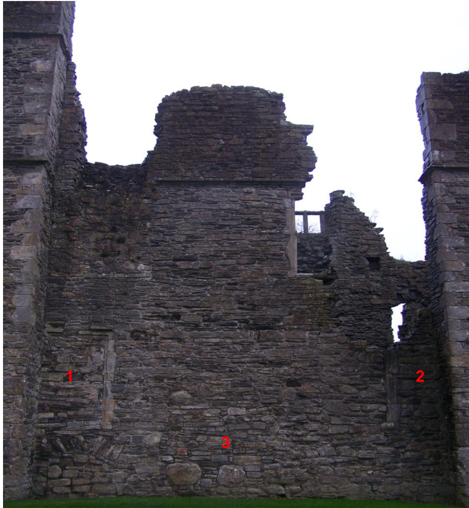
Plate 4 (left): Centre of south-eastern façade showing blocked-up windows (1 & 2) and possible central doorway (3), looking north-west, and Plate 5: Blocked-up doorway on interior side of south-eastern wall of main block, looking south-east
