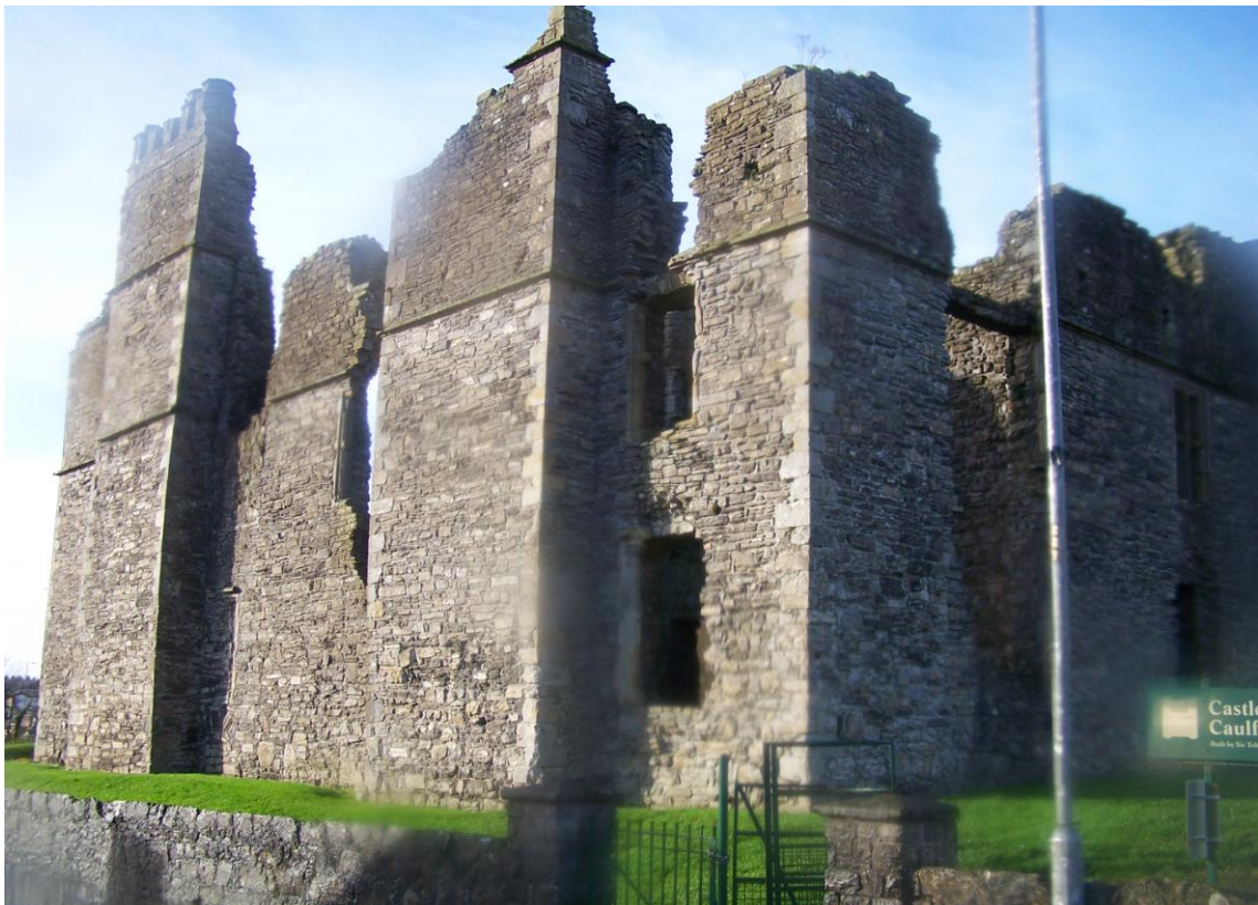
Plate 1: general view of the castle, looking west
