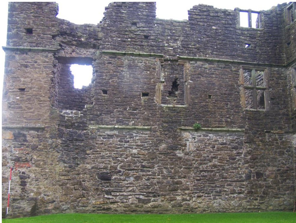
Plate 14: South-western wall of the north-eastern wing, looking north-east
