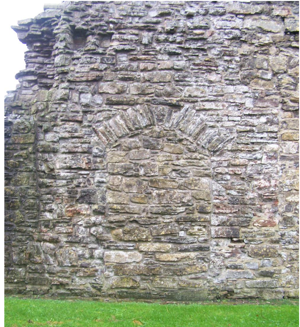
Plate 4 (left): Centre of south-eastern façade showing blocked-up windows (1 & 2) and possible central doorway (3), looking north-west, and Plate 5: Blocked-up doorway on interior side of south-eastern wall of main block, looking south-east
