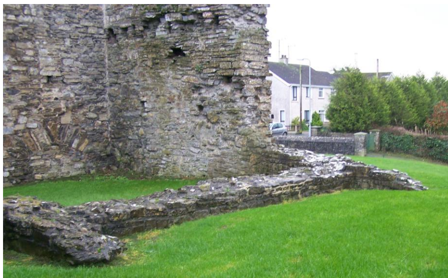
Plate 17: Footings of the south-western wing, looking south
