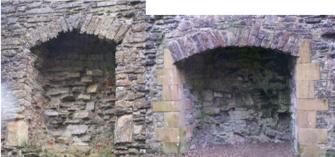
Plate 15 (left): Original first floor fireplace in the north-eastern wall of the north-eastern wing, looking north-east, and Plate 16: Reconstructed ground floor fireplace in the north-eastern wall of the north-eastern wing, looking north-east
