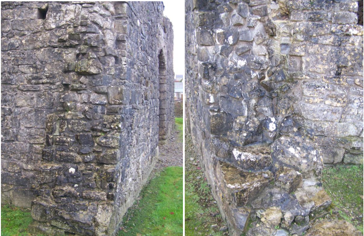
Plate 29 (left): Bawn wall stump at eastern corner of gatehouse, looking north, and Plate 30: Bawn wall stump at northern corner of gatehouse, looking east.
