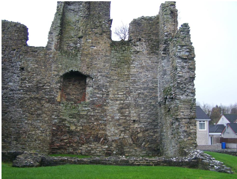
Plate 18: View of the footings of the south-western wing, looking south-east
