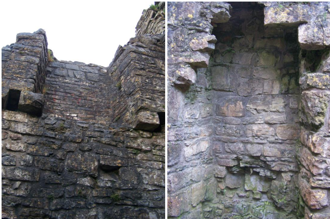
Plate 25 (left): Brick-lined first floor fireplace in the south-eastern room of the gatehouse, looking south-east, and Plate 26: Remains of ground floor fireplace in the north-western room of the gatehouse, looking north-west
