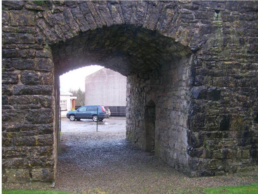
Plate 21: The vaulted passageway through the gatehouse, looking north-east
