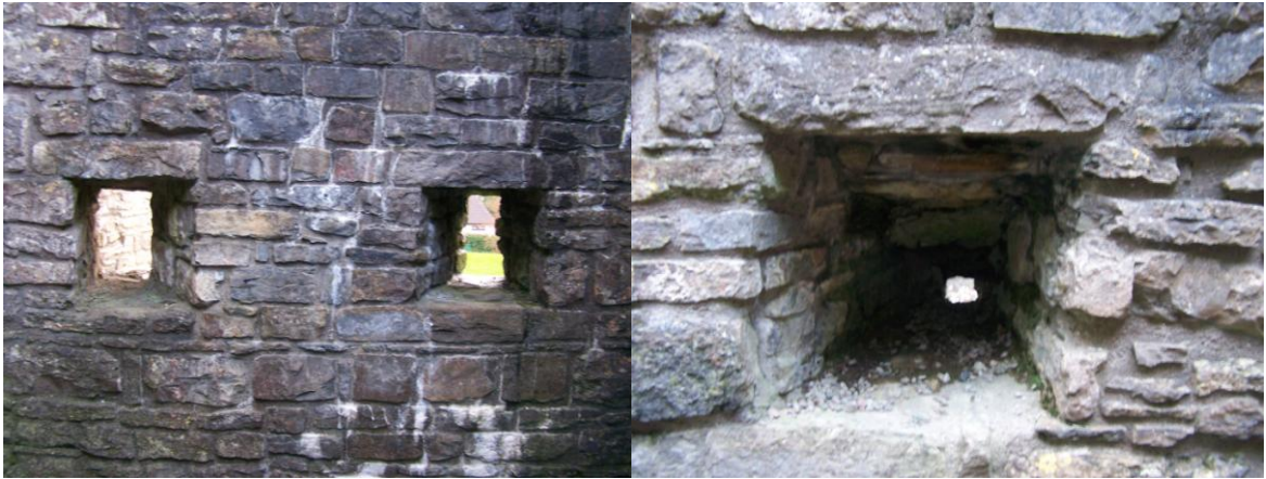
Plates 23 and 24: Possible musket loops in the north-eastern ground floor room of the gatehouse
