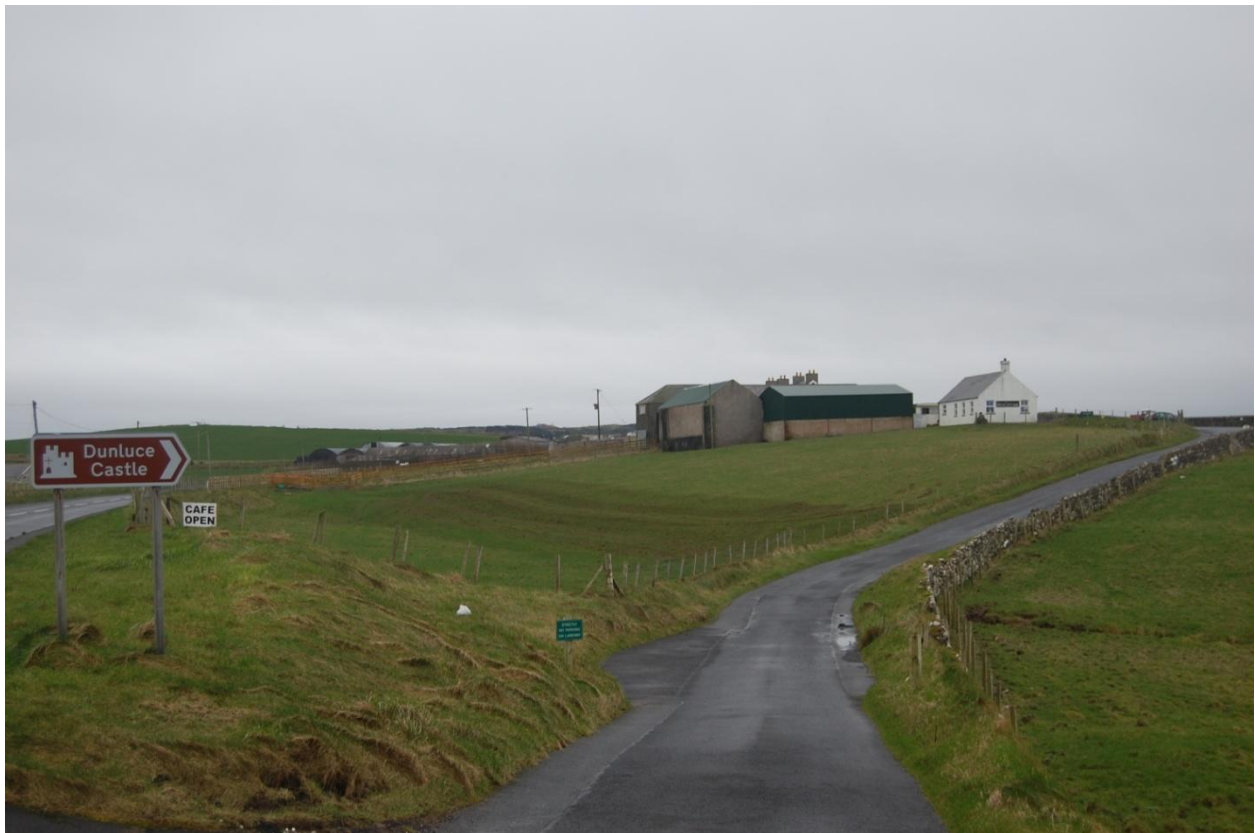
Plate 3. View of Area 2, with Dunluce House and probable 18 th -century barn in the background, facing south-west, from the northern junction of the Castle Road and Dunluce Road.
