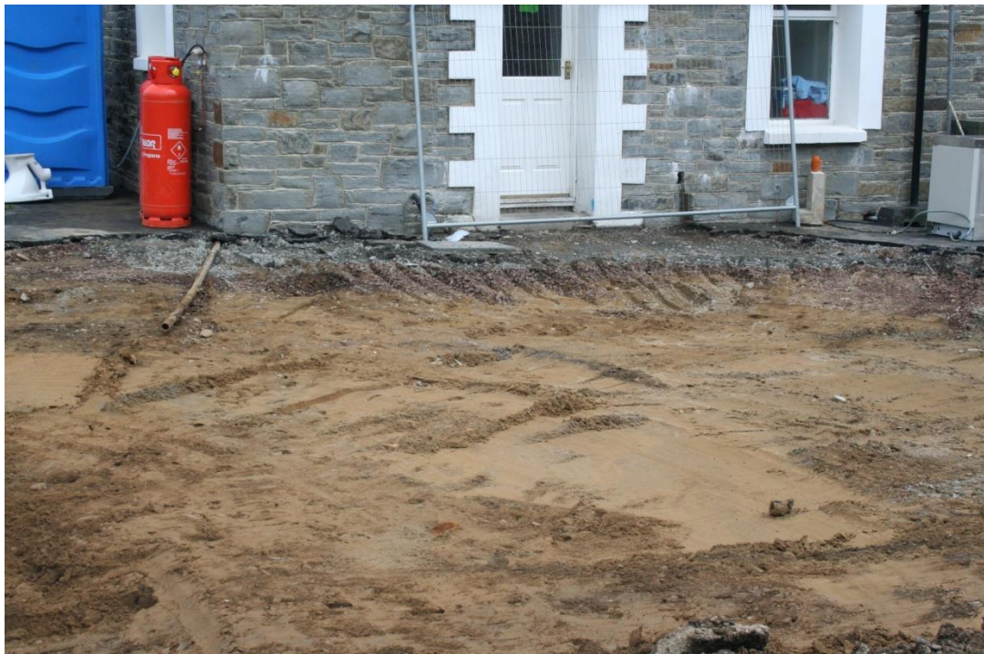
Plate 10: Driveway area on removal of tarmac and hardcore layer (C102), showing natural sand subsoil, looking east.
