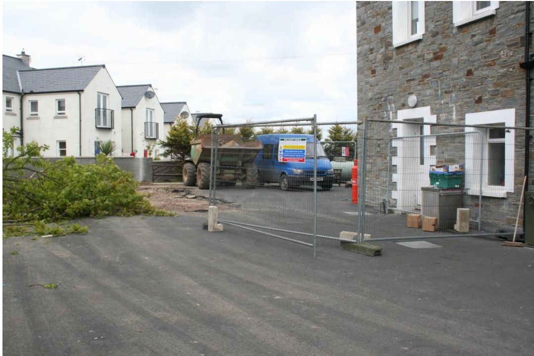
Plate 9: Tarmac area, between the garden and the nursing home, looking north.
