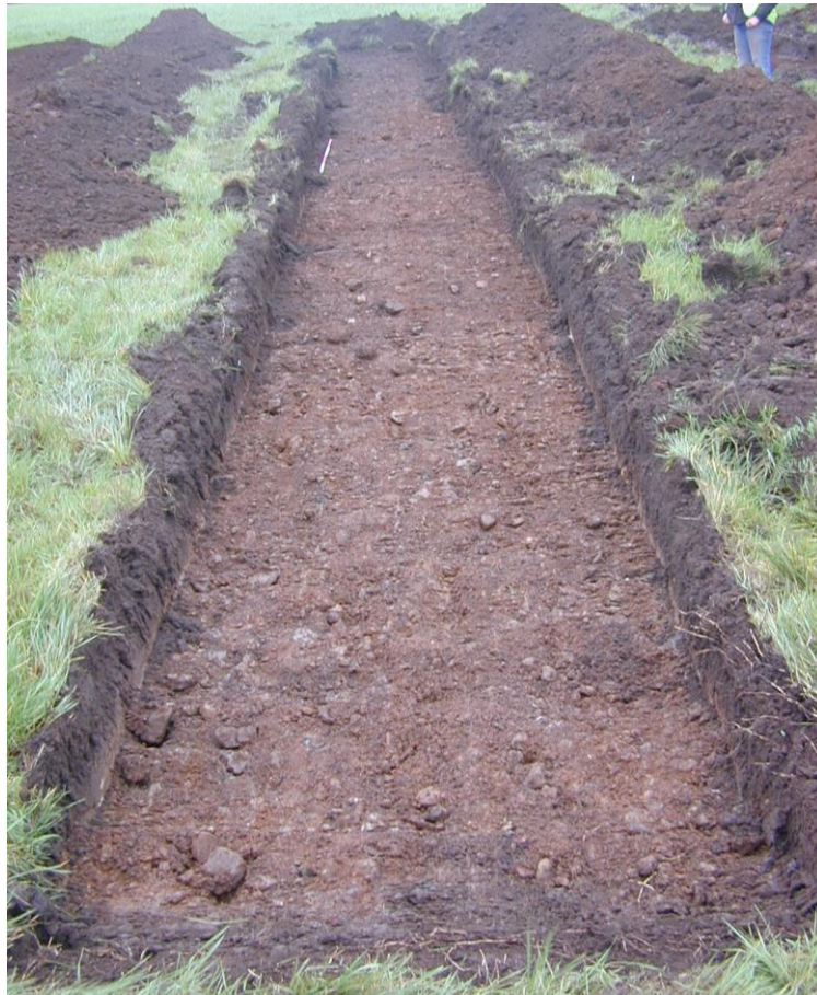
Plate 4: General view of Trench 2 looking east southeast.
