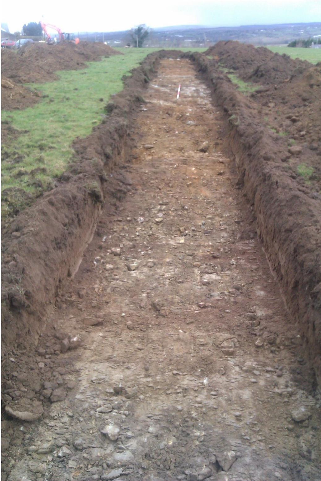
Plate 9: Trench 3 following excavation to subsoil level, looking north-west
