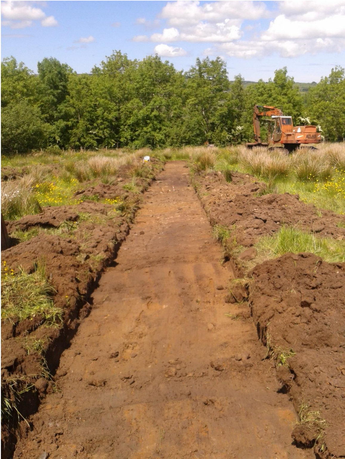
Plate 12: Trench 2 following excavation to subsoil level, looking north
