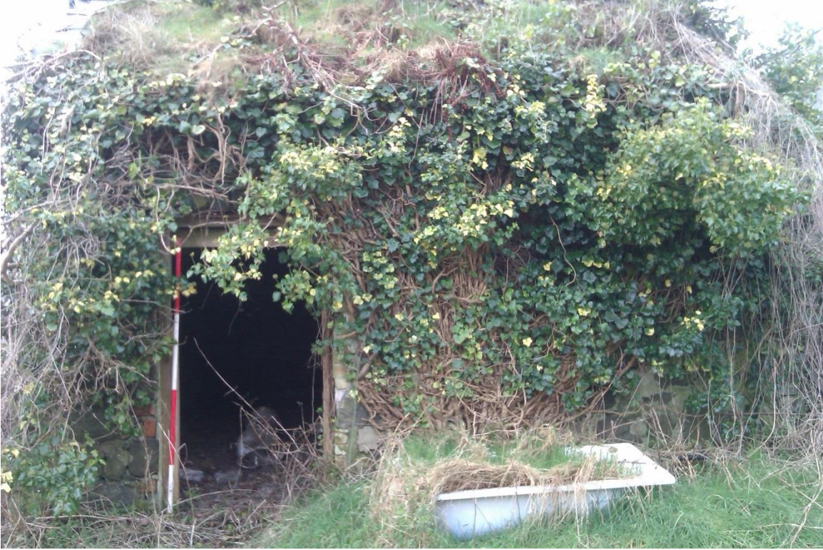
Plate 7: View of building 2, looking west
