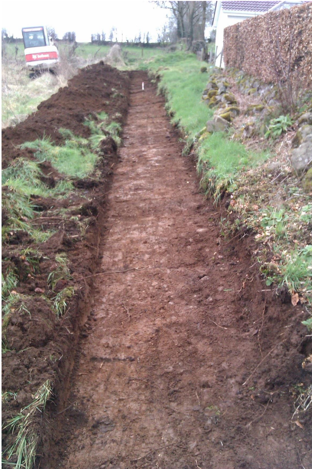
Plate 11: Trench 1 following excavation to subsoil level, looking north
