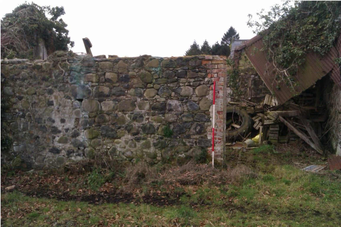
Plate 9: Building 3, looking west
