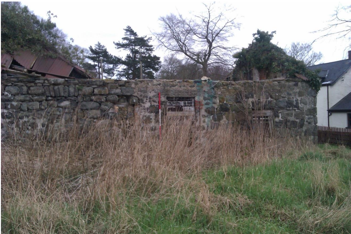
Plate 8: Building 3, looking east
