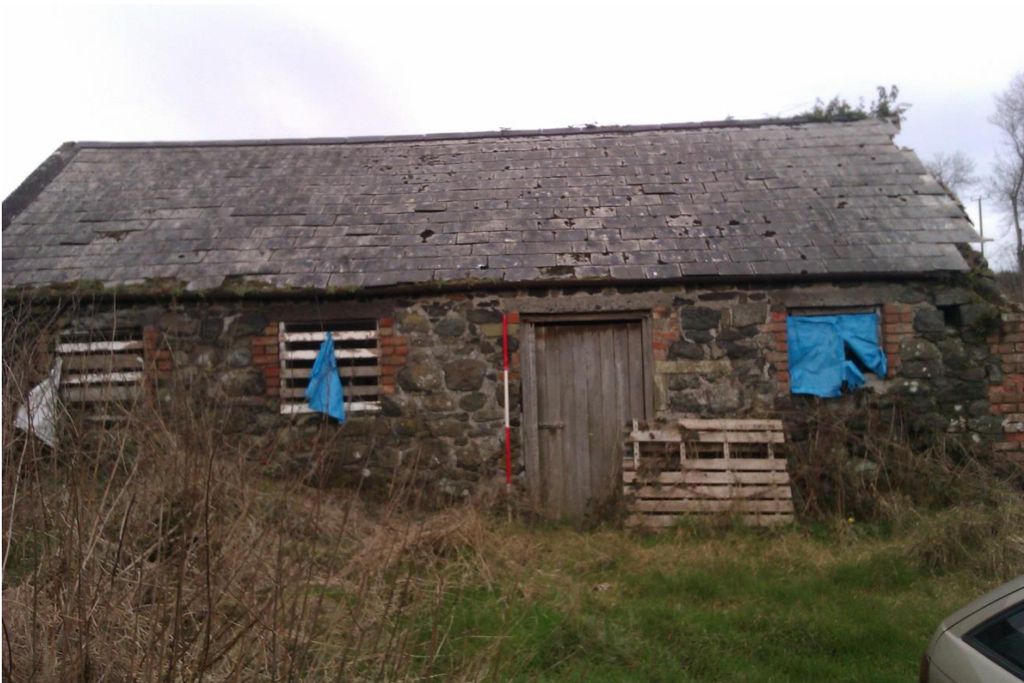
Plate 6: View of building 1, looking north
