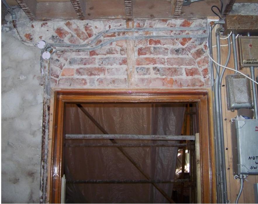
Plate 7: Bricked up archway above interior entrance from tower to doorway
