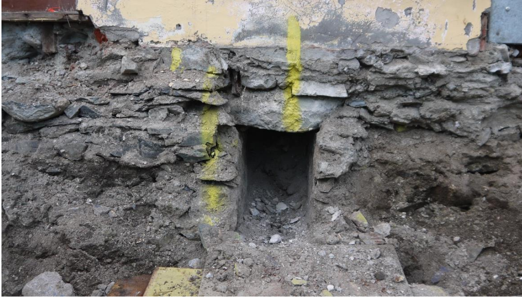
Plate 6: Air vent below the floor level in the eastern gable
