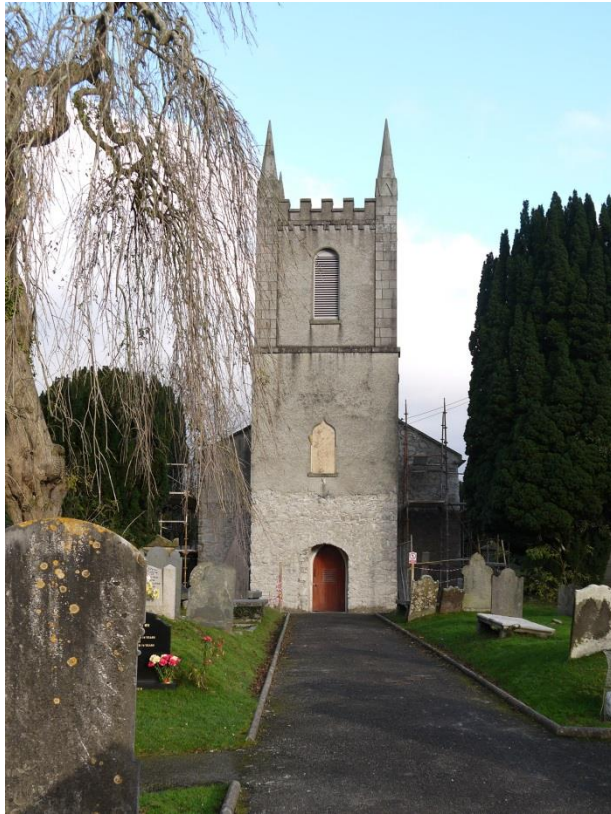
Plate 4: Tower looking east
