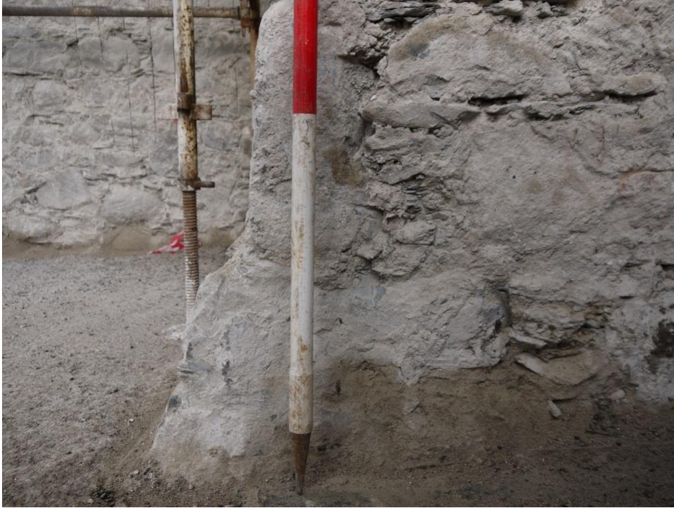
Plate 3: Slight base batter at south-west corner of church
