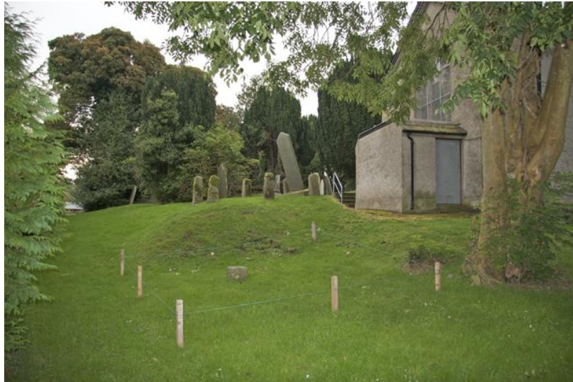
Plate 2: Previous vestry room looking south-west
