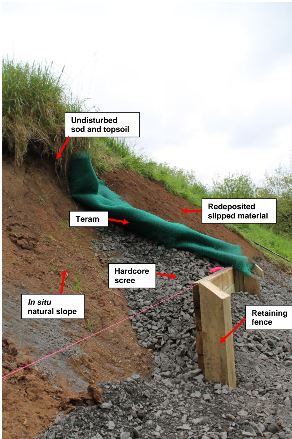
Plate 4: Detail of the consolidation works, looking west.
