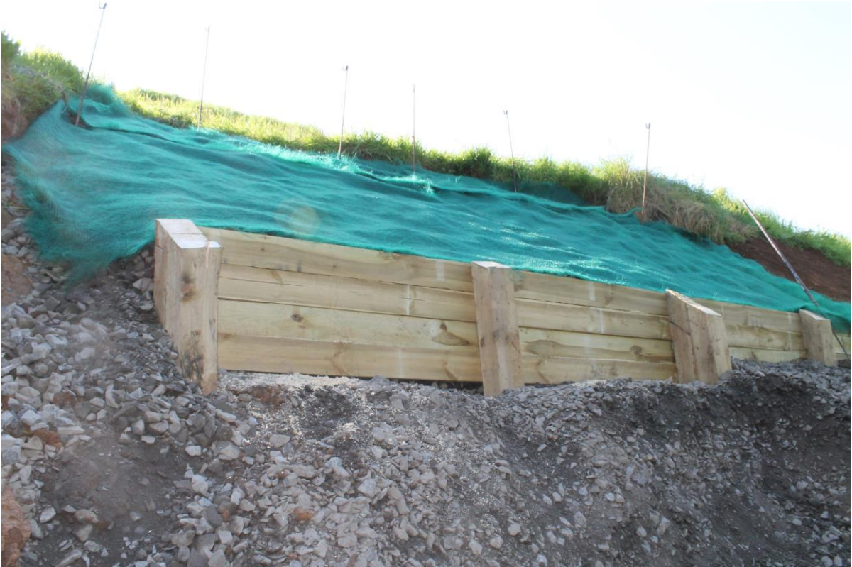
Plate 3: Construction of the 'upper tier' of the retaining fence, looking south.
