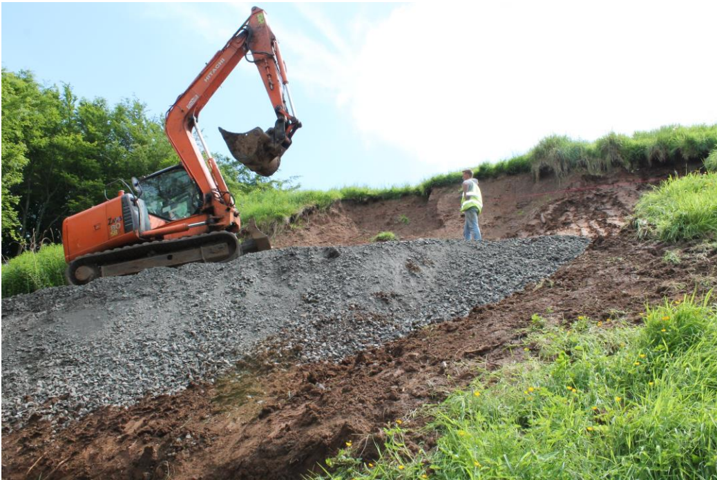
Plate 2: Mechanical removal of the slipped material, looking south-east.
