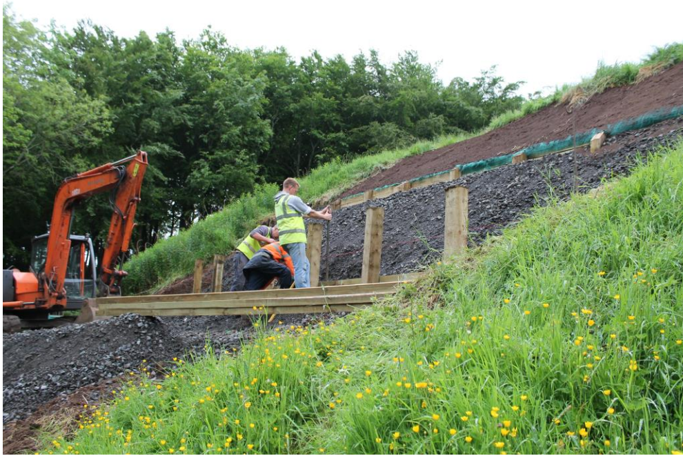
Plate 5: Construction of the second retaining fence, looking south-east.
