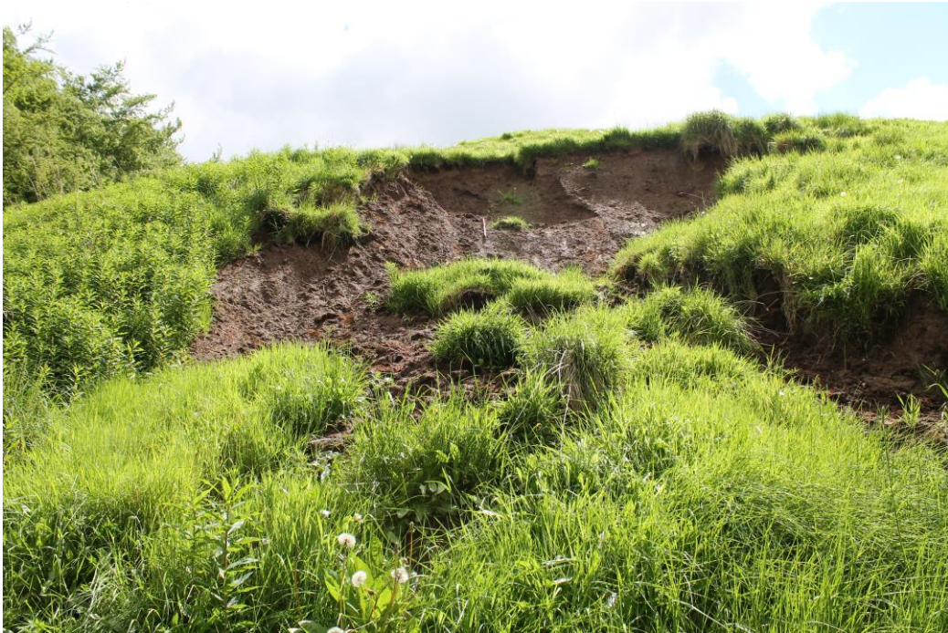
Plate 1: Slippage prior to the consolidation works, looking south-east.
