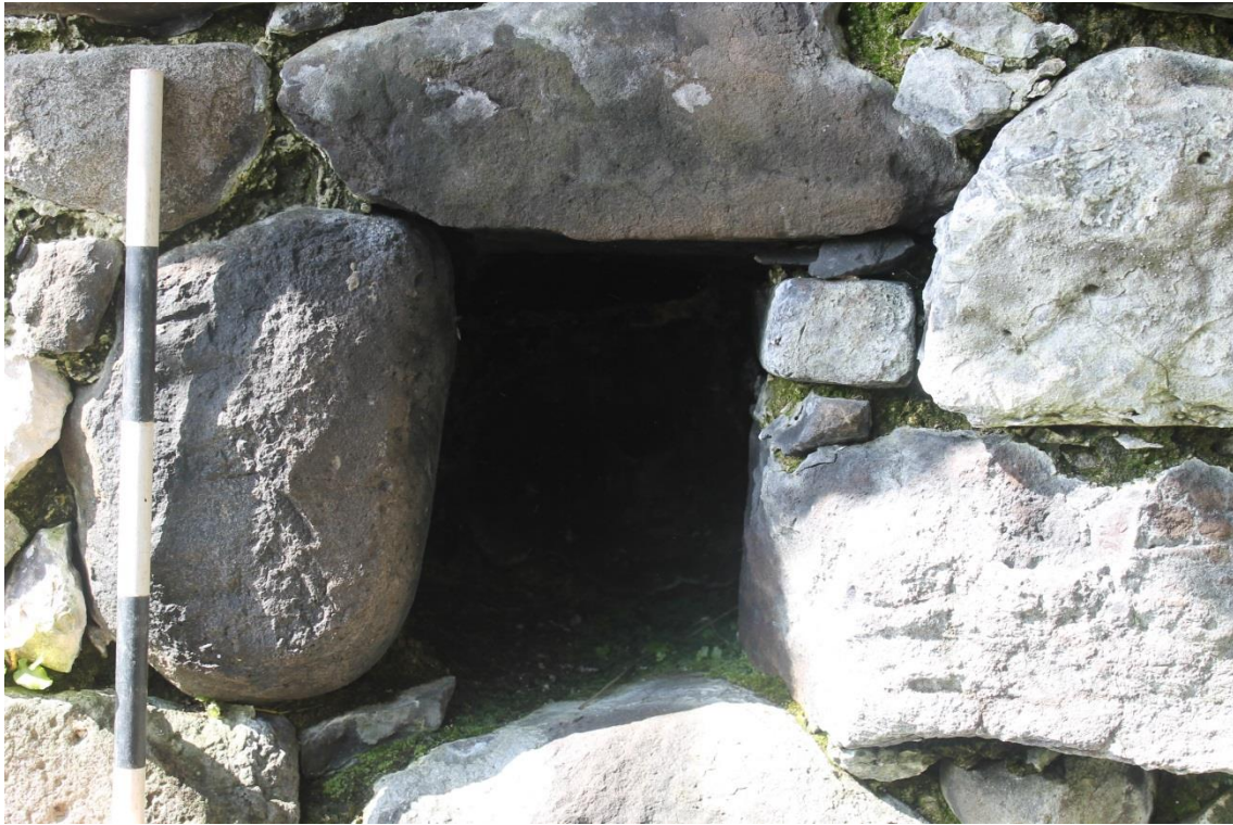
Figure 16: Cavity in the southern wall of the recess, looking south.
