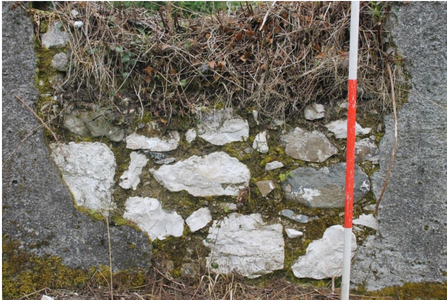
Figure 10: Lime and basalt in front façade of the vernacular house.
