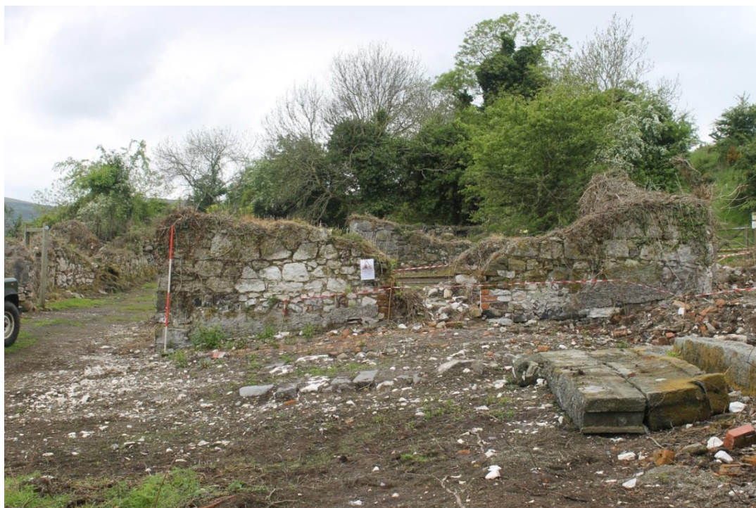
Figure 12: Cow shed, looking south west.
