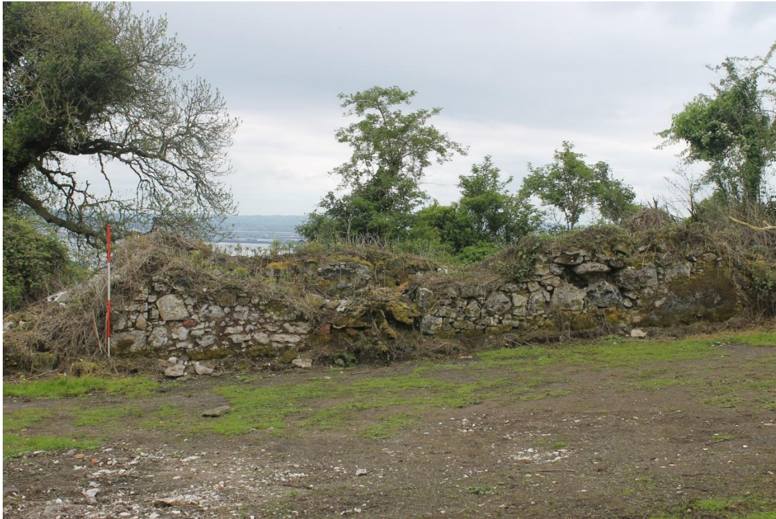
Figure 13: Hay barn, looking south south east.
