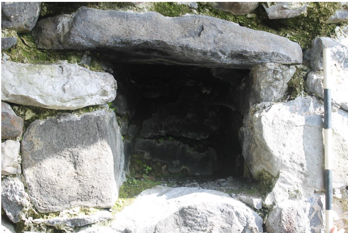
Figure 15: Cavity in the northern wall of the recess, looking north.
