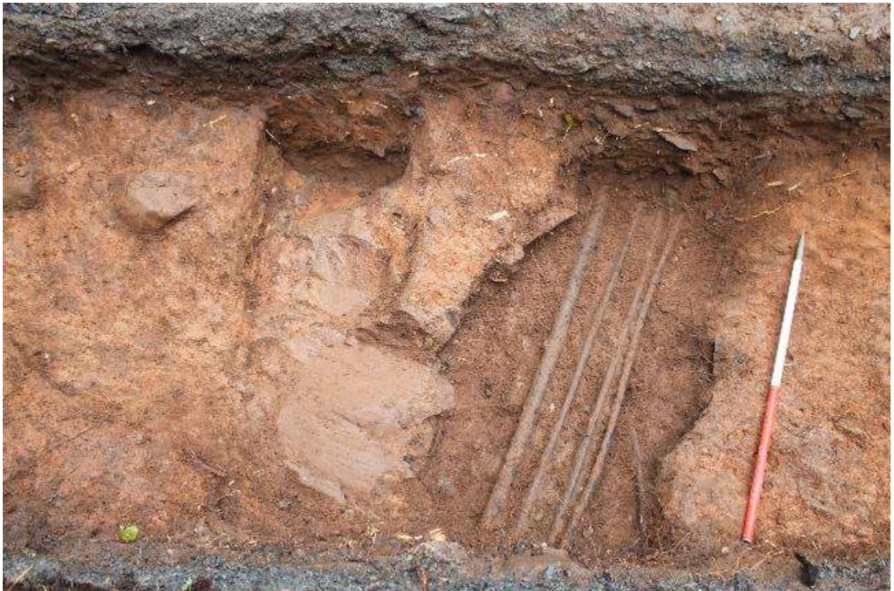
Plate 18. Trench 2 from the East. Detail of the two service trenches (C. 216 and C. 213) and the service cables (C. 211).
