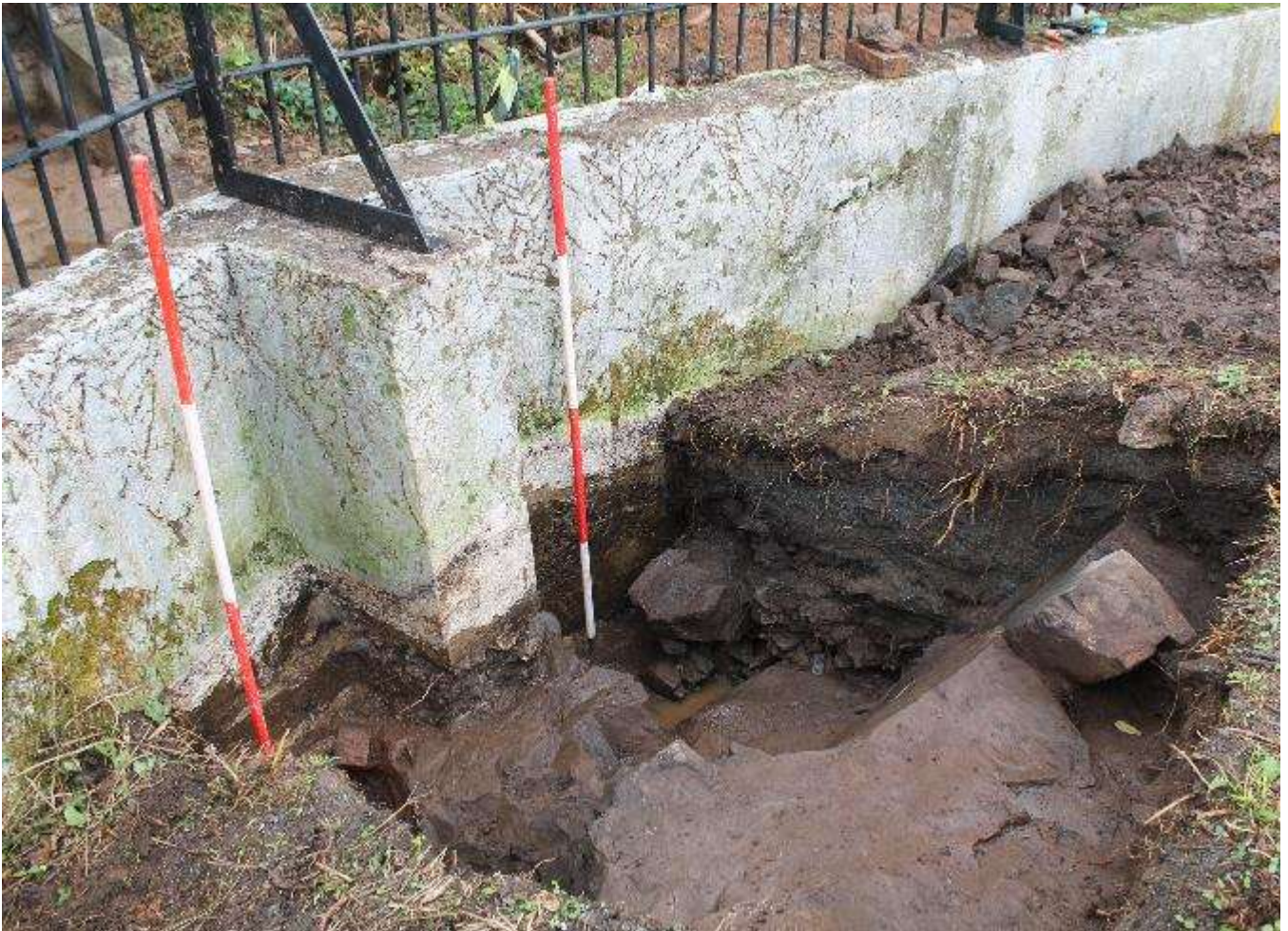
Plate 15. Trench 1B, Northern Extension. West-facing section showing the later stone perimeter wall of the Fort founded on the concrete lintel and layers of poured concrete. The drop in bedrock where this has been removed is very visible as are the later dumped layers of gravel and sand.
