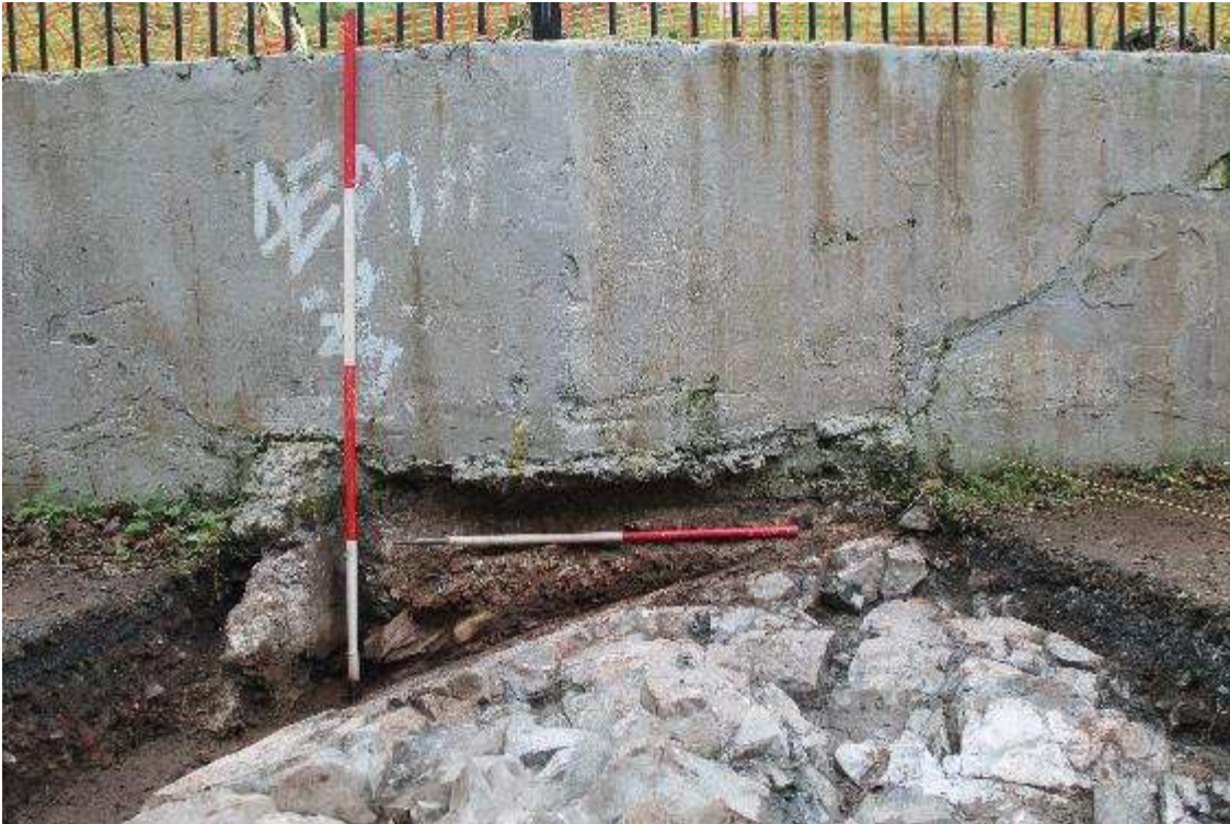
Plate 9. Trench 1A. The southern end of trench showing the stumps of the western and eastern walls of the Blockhouse and the later northern stone perimeter wall (C.1029) of the Fort built over these. Between the Blockhouse walls layers of poured concrete and a concrete lintel were used to level up the uneven bedrock and provide a firm base for the perimeter wall.
