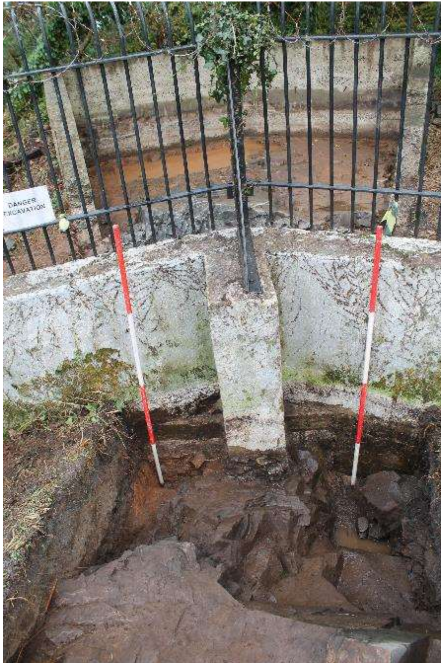
Plate 14. Trench 1B, Northern Extension. South-facing section, showing the later stone perimeter wall of the Fort founded on the concrete lintel and layers of poured concrete and the drop in bedrock where this has been removed. In the background of the shot is Trench 1A/ the concrete Blockhouse over which the stone perimeter wall had been built.
