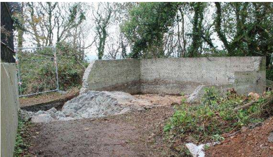
Plate 10. Trench 1A. The fully excavated Blockhouse from the south-west. At the far left of the shot the later northern stone perimeter wall of the Fort is visible. Also visible are the modern gravel path and the section of bedrock and the sections of the western and eastern walls of the Blockhouse which had been removed to facilitate the creation of the path.
