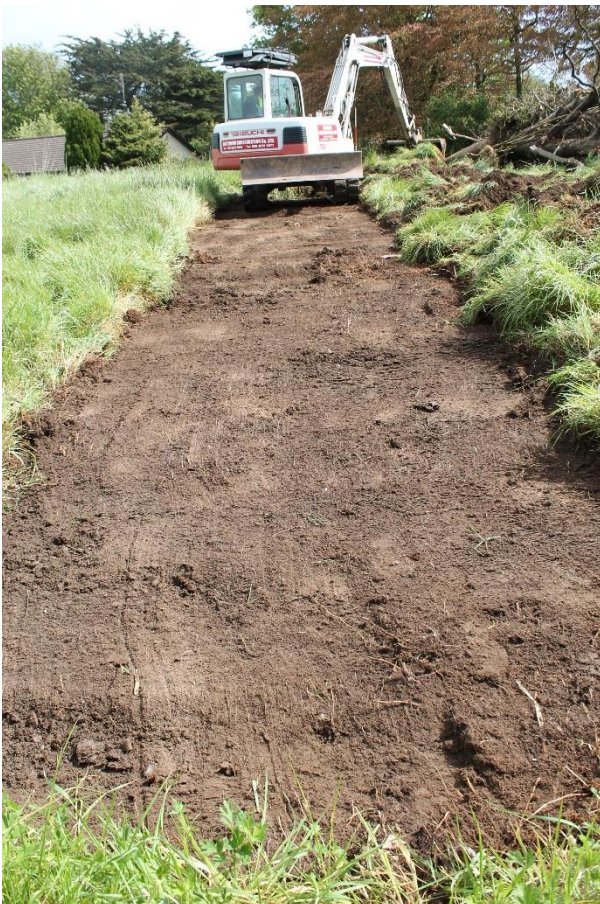
Figure 8: Trench 1, post-removal of sod layer C101, showing topsoil layer C102.
