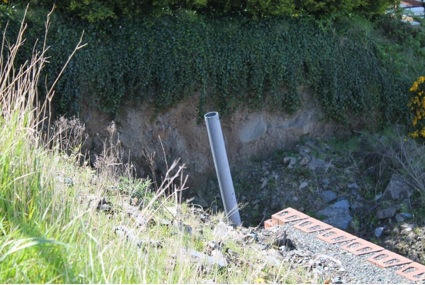
Figure 19: View from northern end of site (to remain undeveloped). Looking west towards cut-away, developed ground beyond the development area. Sterile clay and bedrock is visible throughout the exposed section. Difference in ground levels is approximately 6m.
