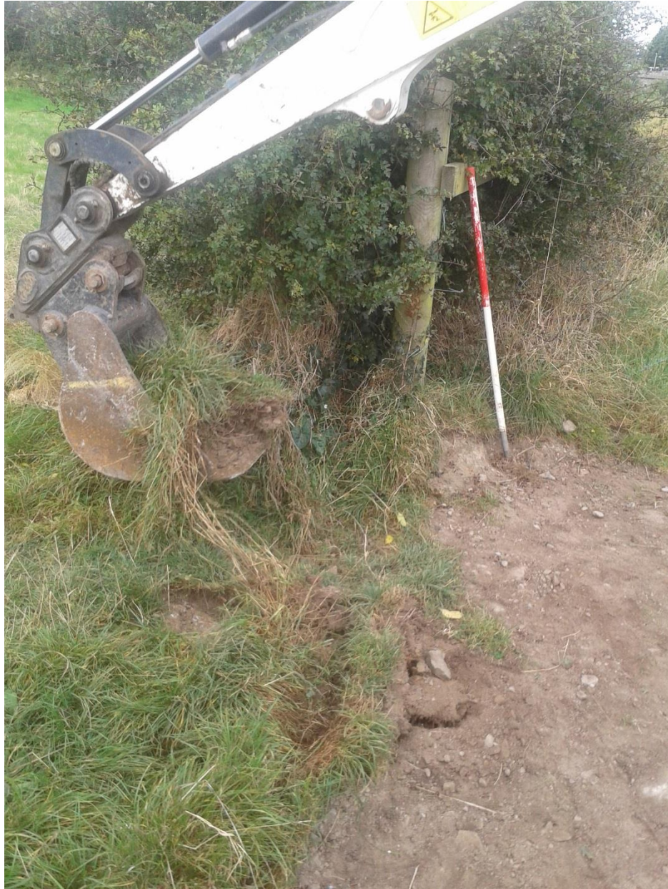
Plate Two: Monitoring the gate installation at Point B, looking west
