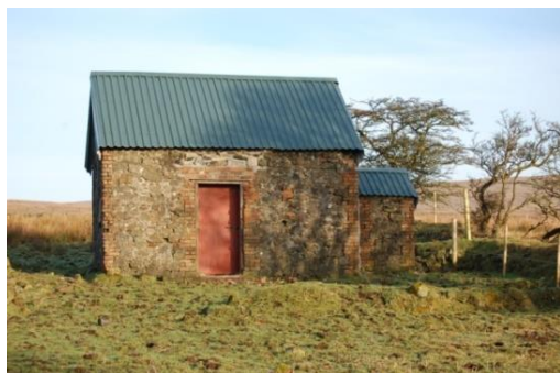
Pl 8 Outhouse viewed from the south
