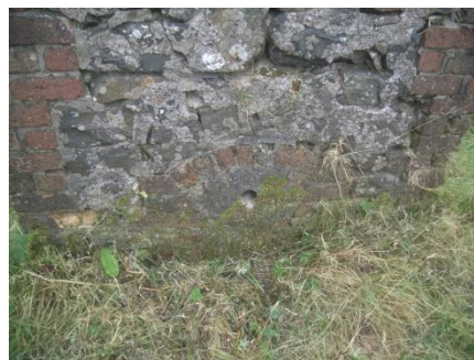
Pl 9 Blocked opening in east wall of outhouse projection
