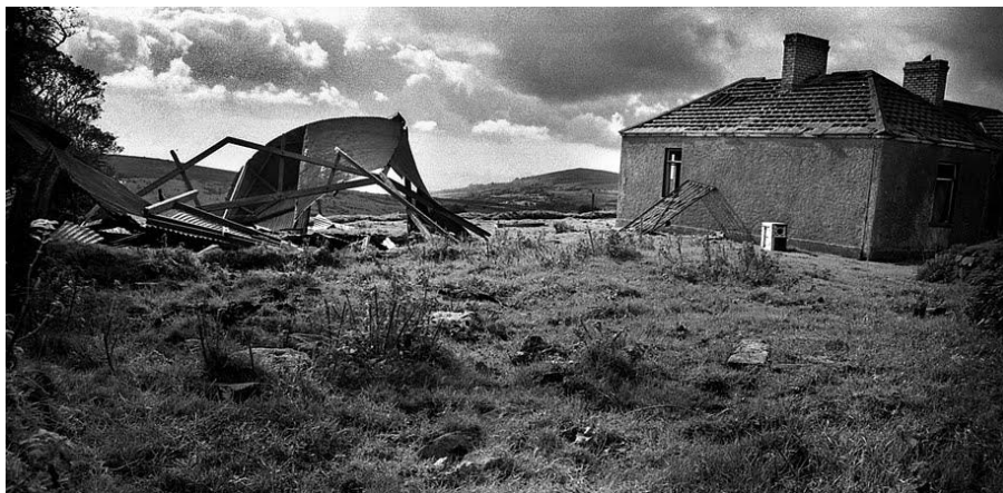
Pl 2 Divis Lodge viewed from north-east, possibly taken in c1968. (NT photographic collection)
