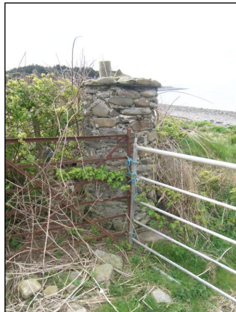
RIMG0062 Gate post at field entrance
