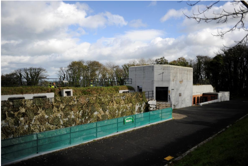
Figure 12: No. 1 Gun Position and magazine, looking north-east
