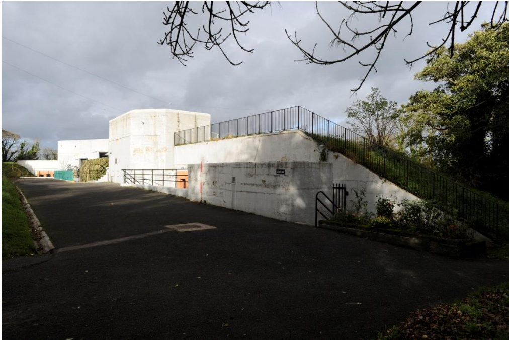
Figure 10: The Gun Battery, looking north-west
