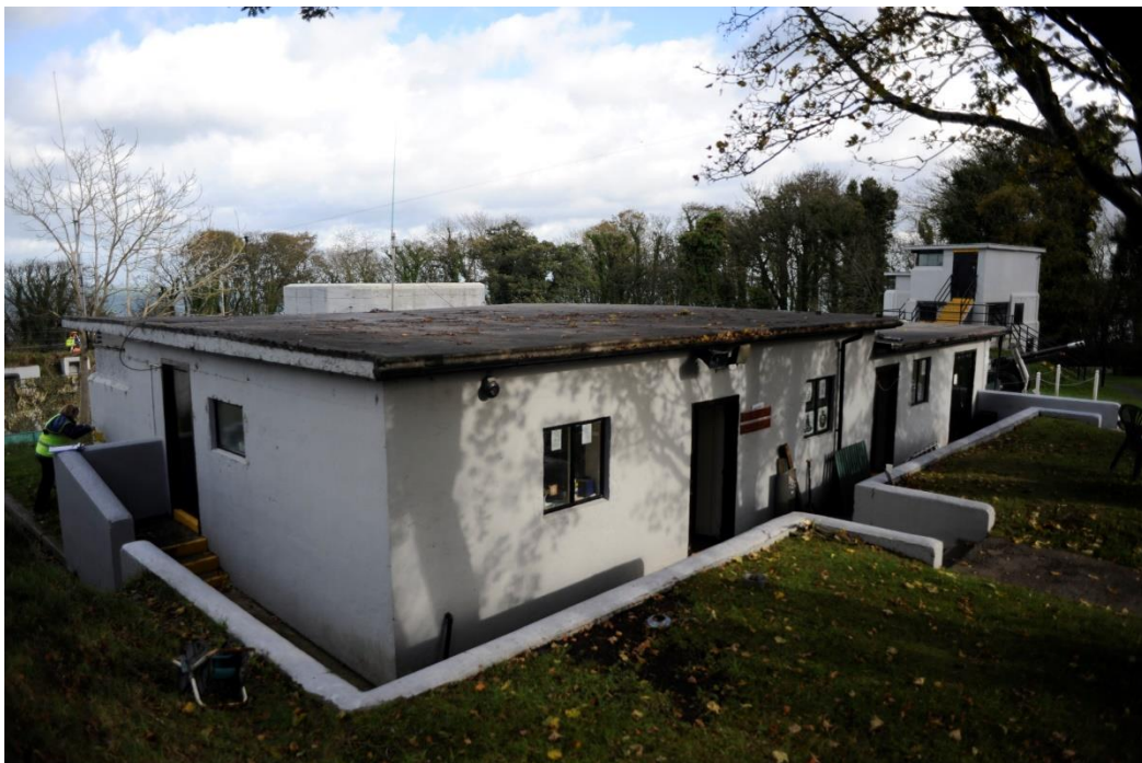
Figure 11: The Fire Command Post, looking north-east
