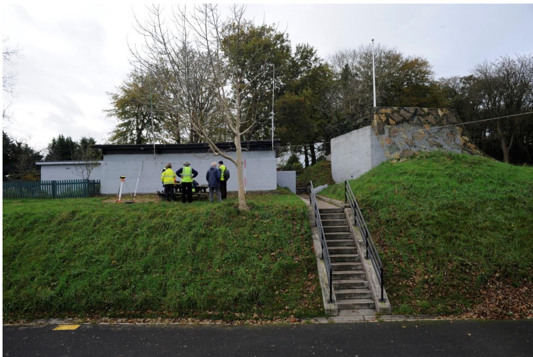
Figure 13: Fire Command Post and Radar Platform, looking south
