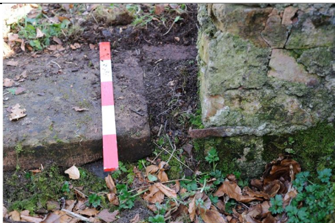
DSC_8686 Detail of doorway
