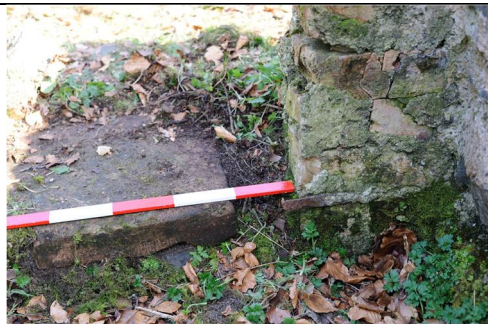
DSC_8685 Detail of doorway
