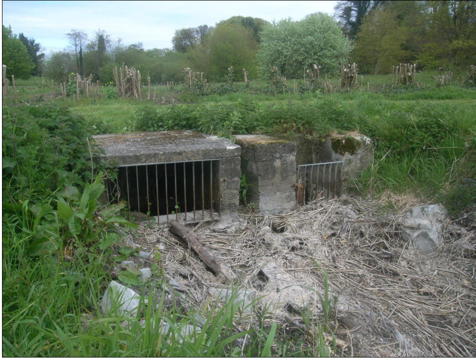
Figure 10: View of eastern drainage sluice, looking east
