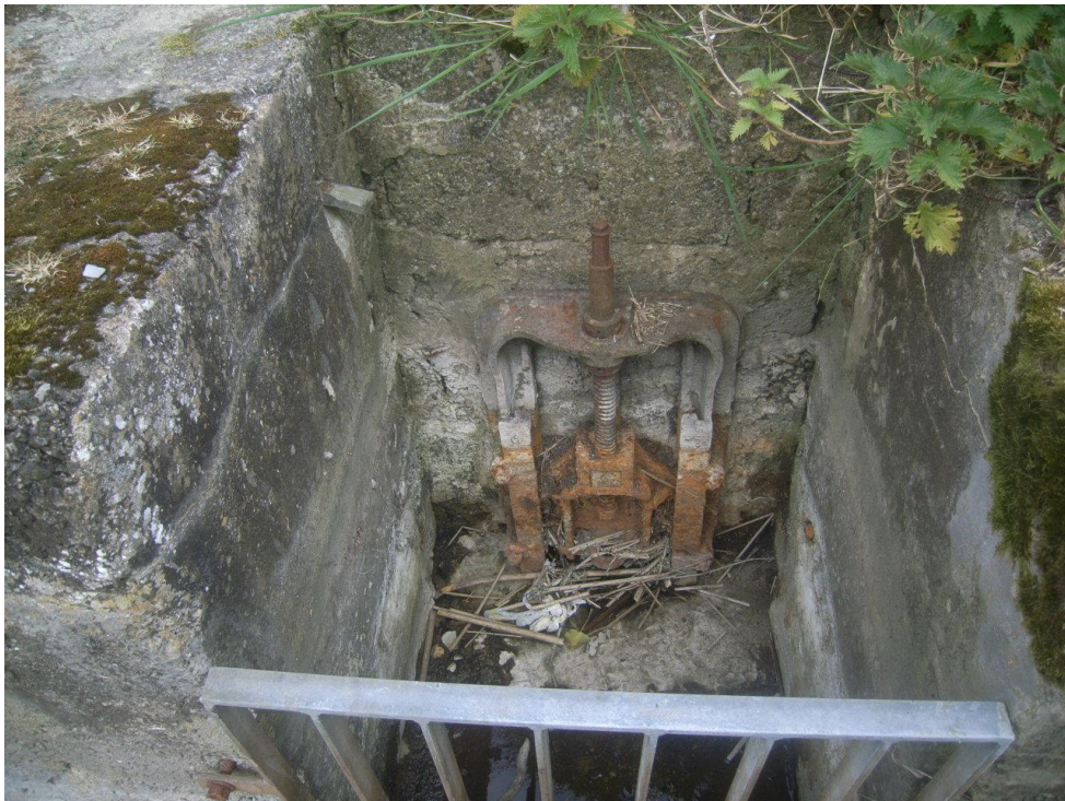
Figure 11: View of eastern sluice gate, looking east
