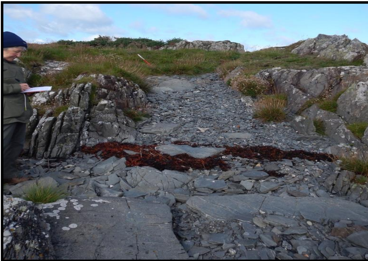
Figure 11: Rough surface on parts of Coach Road, looking north.
