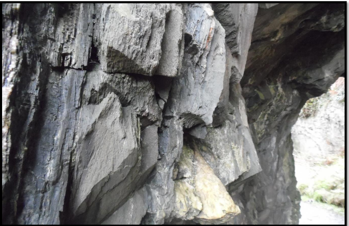
Figure22: Showing chisel marks in tunnel, looking east.
