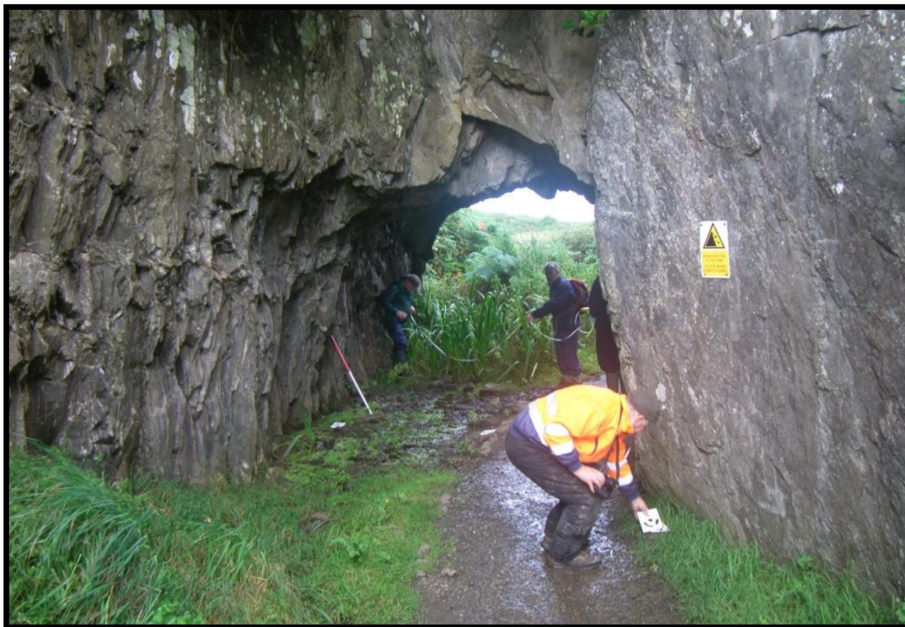
Figure 09: Members of the Survey Team inside tunnel, looking north.
