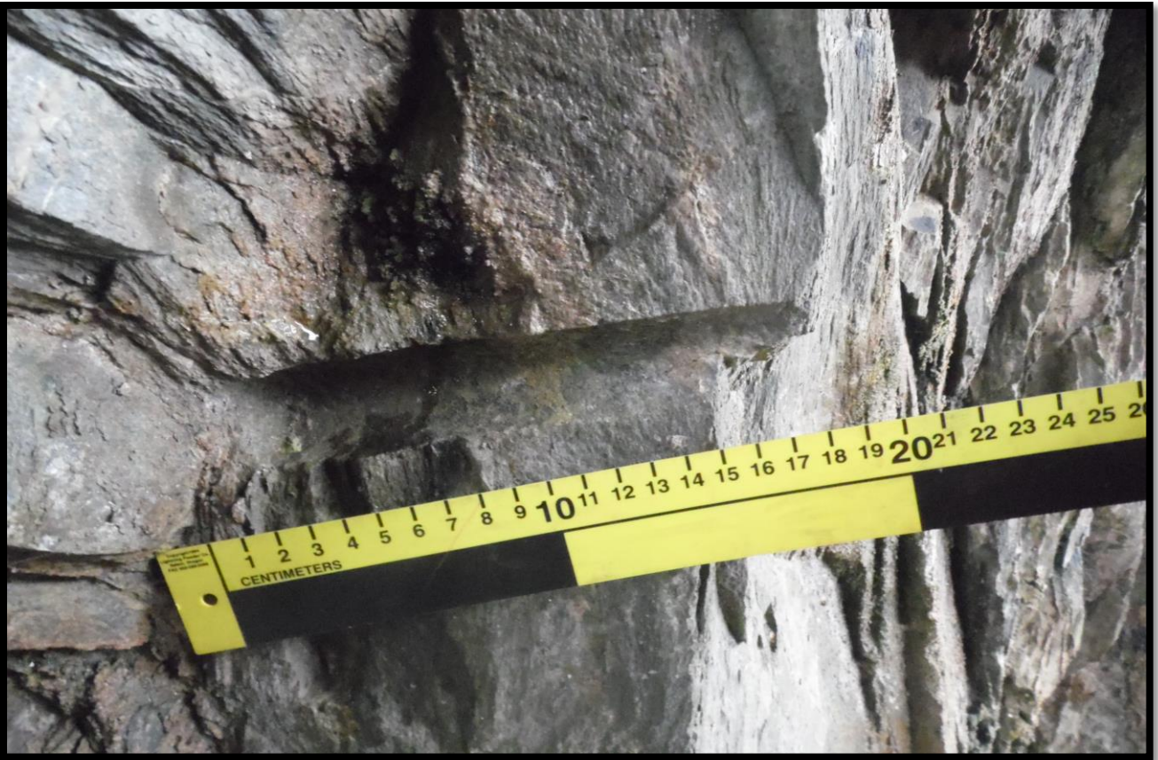
Figure21: Showing drill marks inside the tunnel looking east.
